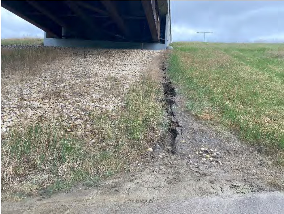
Photo 9: Erosion below the NB abutment on the south slope due to damaged waterproof membrane on abutment. Looking southeast.
