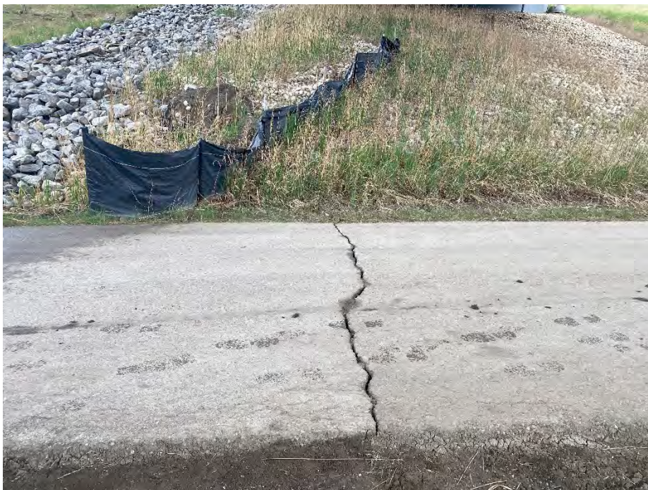
Photo 10: Crack in the paved trail below the NB lane of south abutment. Looking southeast.
