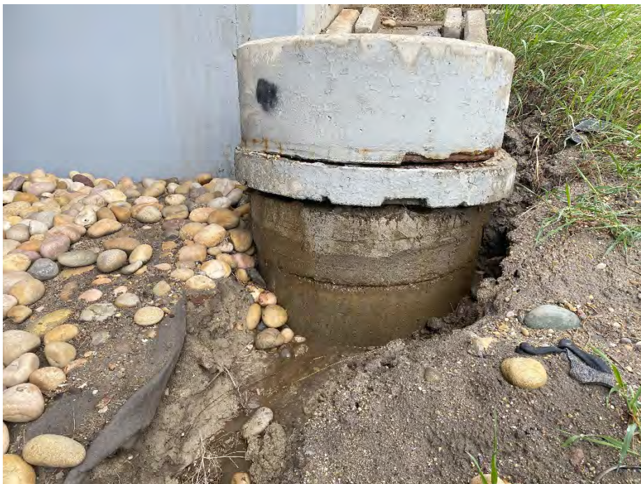
Photo 8: Catch basin on west side of NBL south abutment, not containing flow. Looking southeast.
