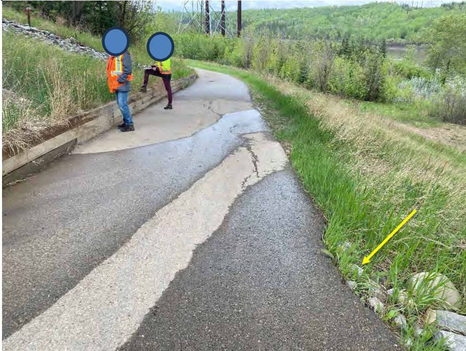
Photo 7: No change to trail crack pattern. Minor loss of trail. Looking northeast.
