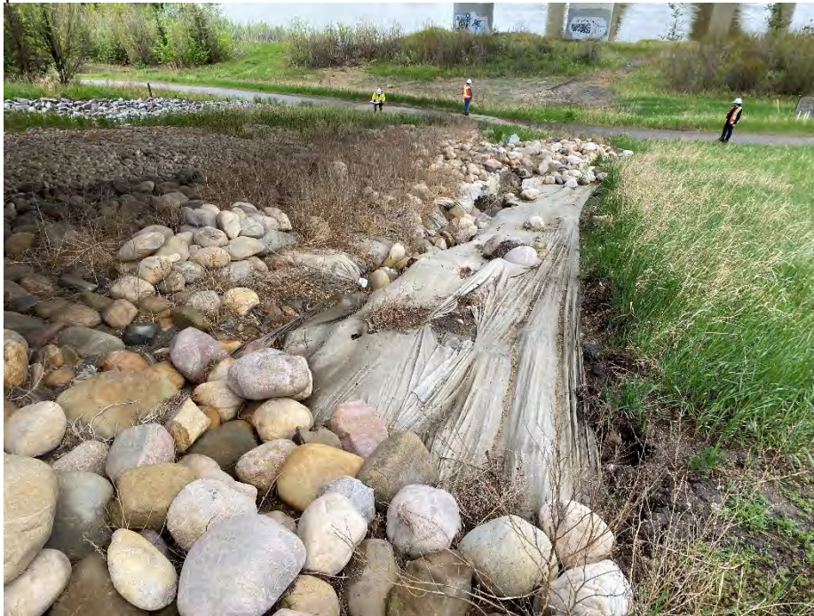
Photo 5: Erosion gully on west edge of riprap on the north bank under the NBL. Looking southeast.
