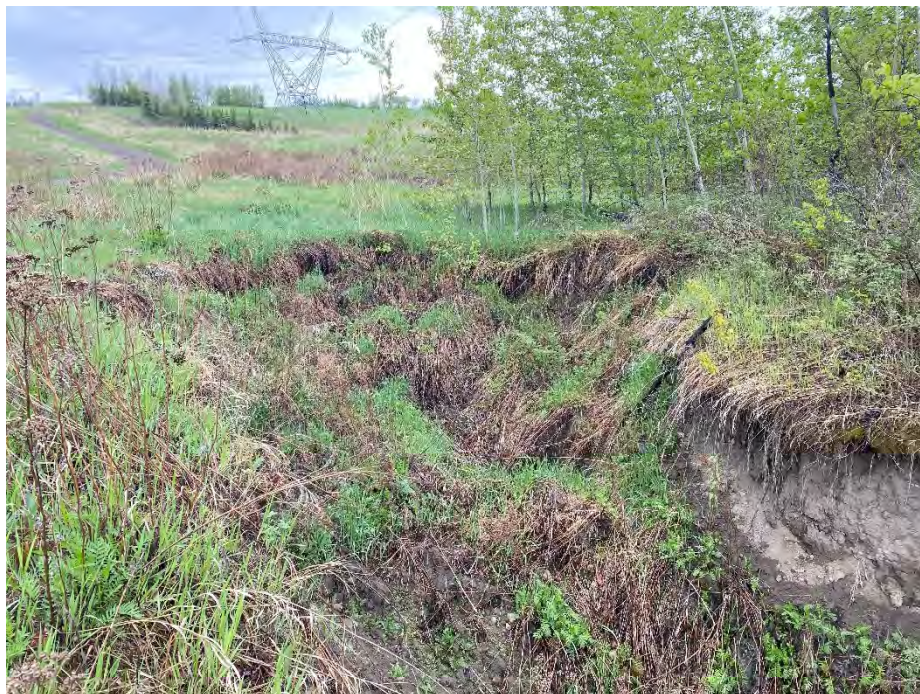
Photo 12: Slump around the outfall on the south bank of the river. Looking southeast.
