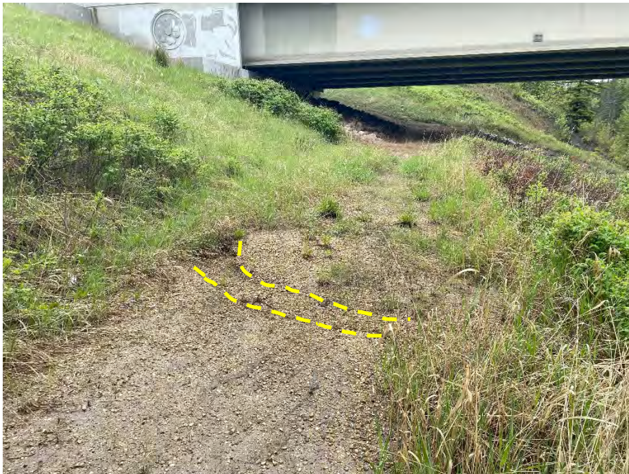
Photo 4: Erosion gully on the footpath between the NW and SW abutments, partially infilled with sand and sediment. Looking northeast.
