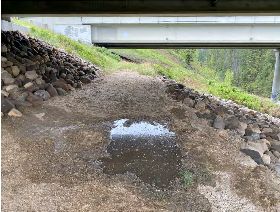
Photo 3: Erosion and ponded water on footpath near NW abutment for SBL. Looking northeast.
