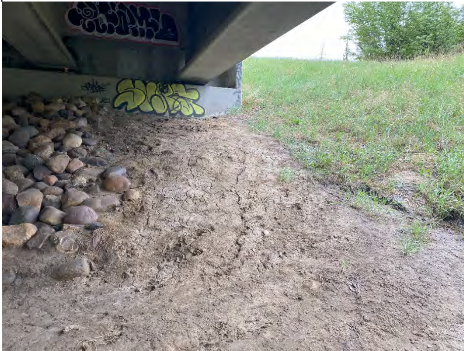
Photo 5: Erosion at the north corner of NW abutment. Looking northwest.
