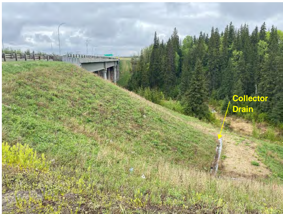
Photo 2: Soil nailed slope at north and south slide area, collector drain installed at toe of repaired slope. Looking southeast.
