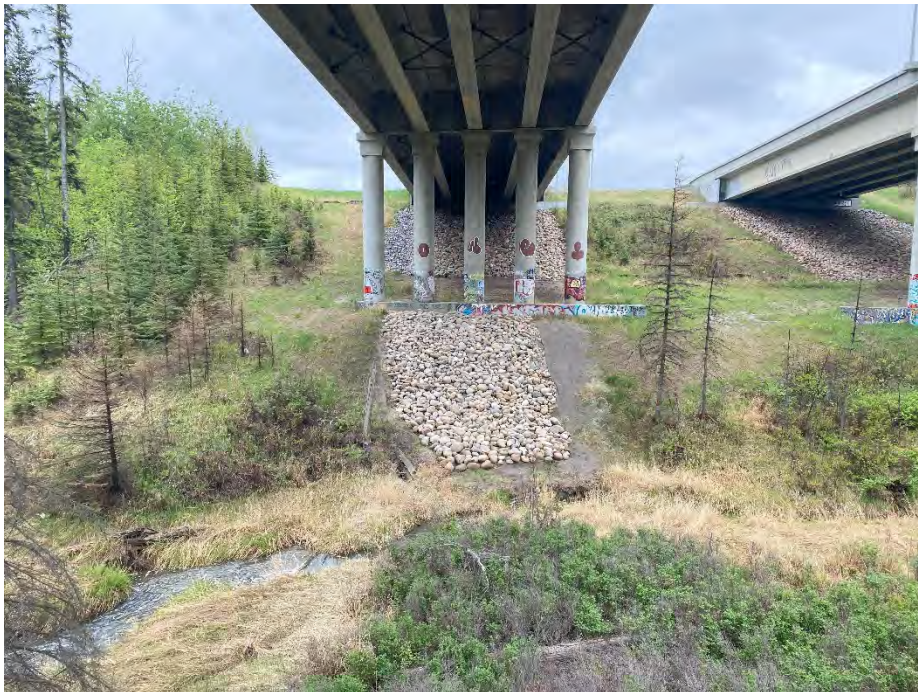
Photo 10: Repaired slope failure on east bank below AHD northbound pedestal. Looking southeast.
