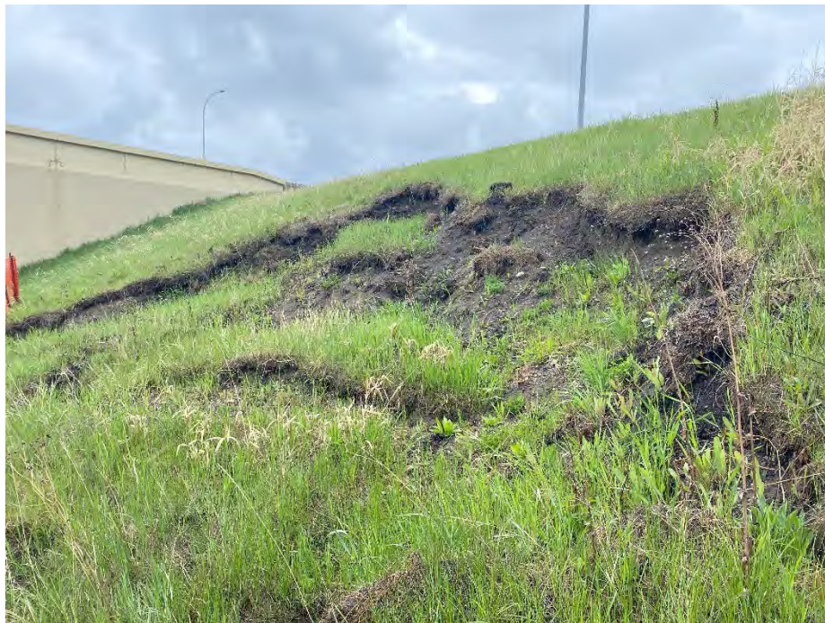
Photo 2: Scarps near top of slump. Looking southeast.
