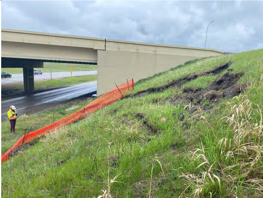
Photo 3: Mid to upper portion of slump with displaced snow fence, looking east.
