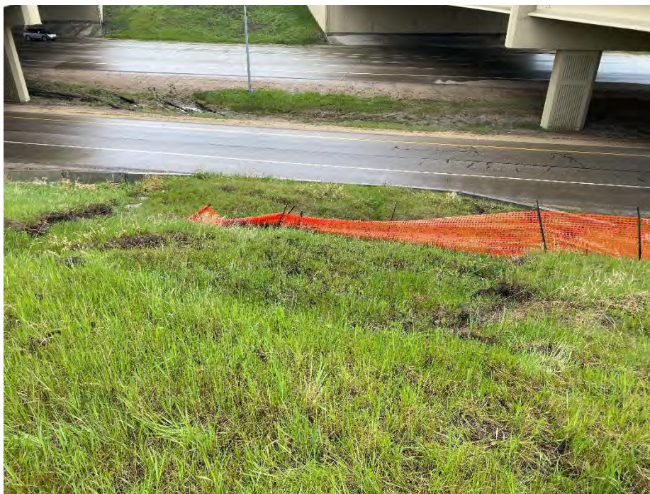
Photo 6: Slumping viewed from the crest of the embankment. Looking north.
