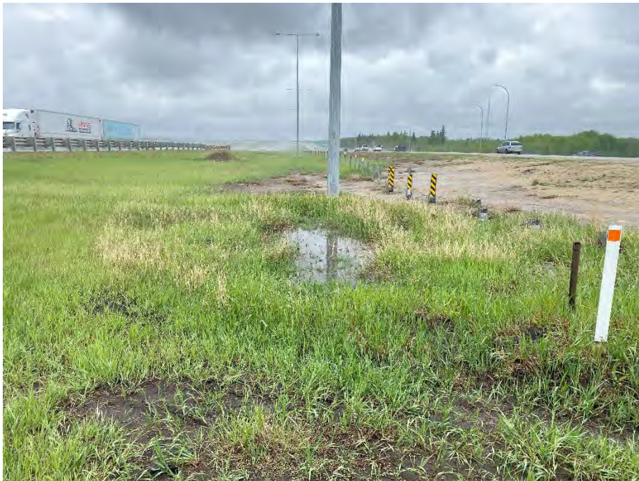
Photo 8: Low area south of embankment crest, ponded water present. Looking south.
