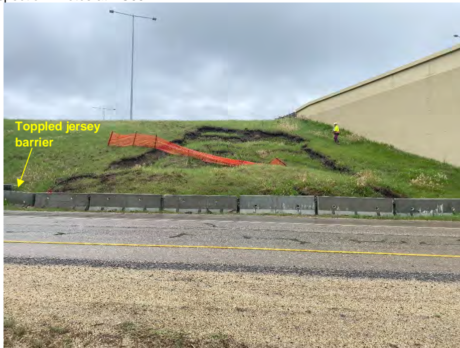
Photo 1: Slump on south embankment. Looking southwest.
