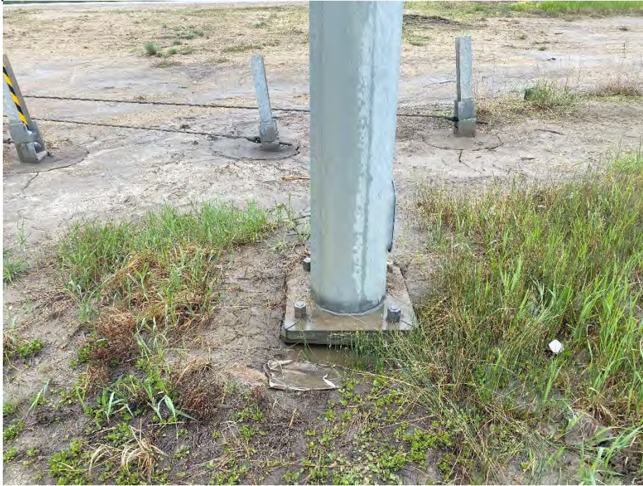
Photo 7: Scouring/settlement of ground around the light standard closest to the embankment. Looking west.
