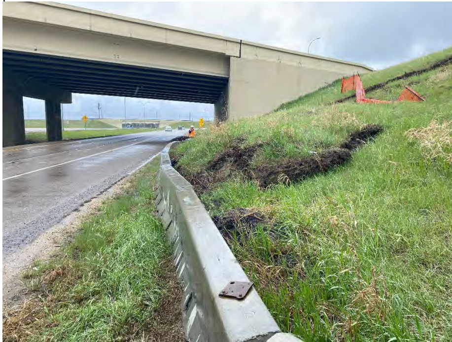
Photo 5: Toe of the embankment/slump. Looking southeast.
