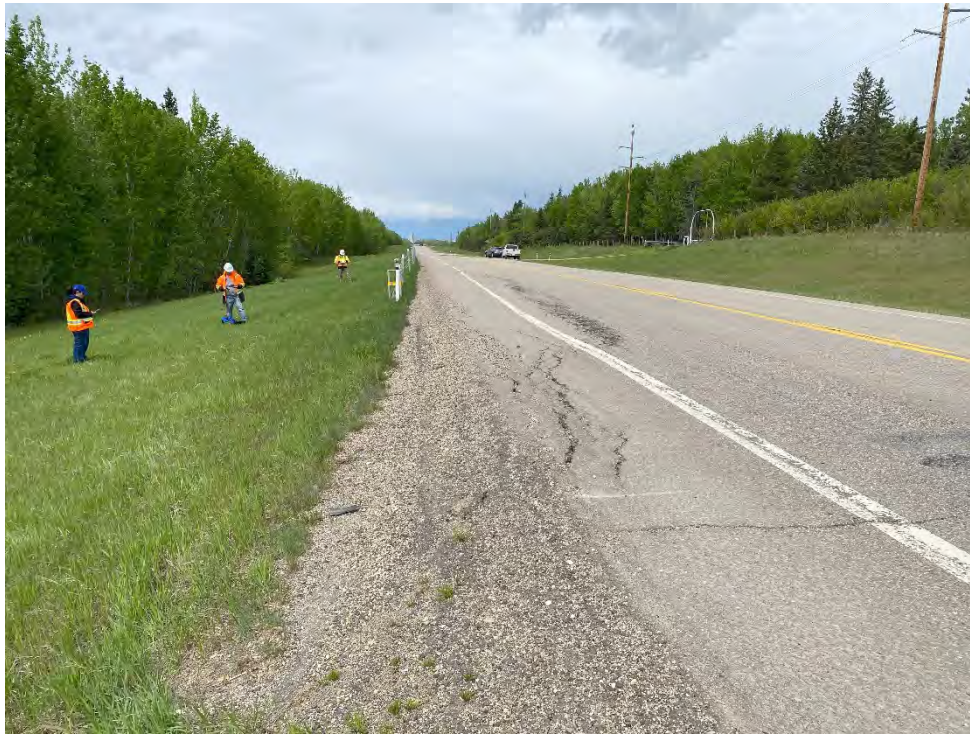
Photo 1: Cracking in the southbound lane, south end. Looking north.
