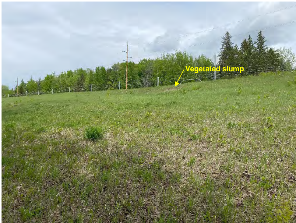
Photo 6: Vegetated slump, looking northeast from tree line.
