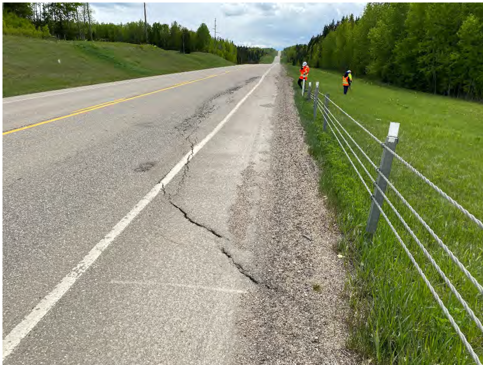
Photo 2: Cracking in the southbound lane, north end. Looking south.
