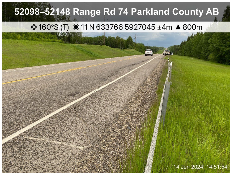
Photo 2: Highway 22 cracking in the southbound lane, north end. Looking south.
