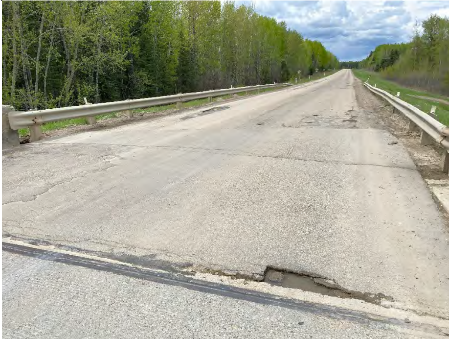
Photo 11: Pavement surface at west abutment with multiple potholes. Looking west.
