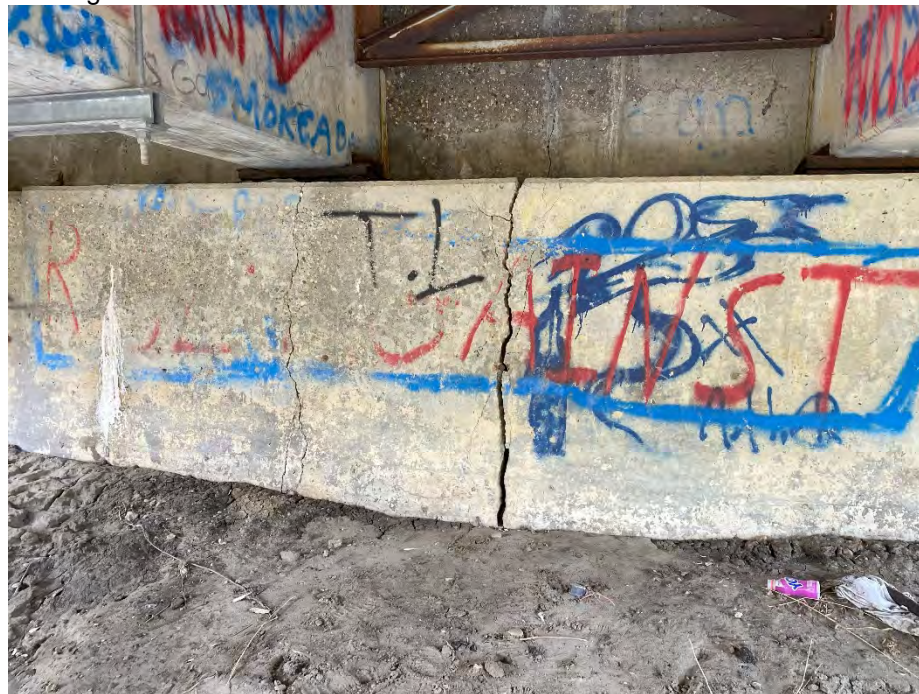
Photo 8: 20 mm crack at west abutment. Looking west.
