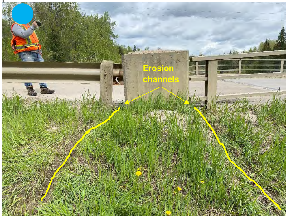
Photo 13: Erosion channels forming off the east bound lane at the west abutment. Looking north.
