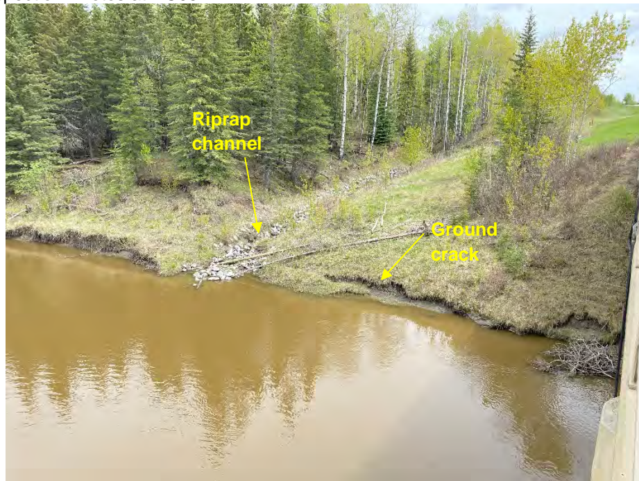
Photo 9: Riprap lined channel and ground crack north of east abutment. Looking northeast.
