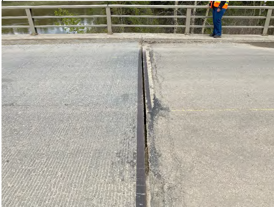
Photo 5: Gap at expansion joint with rubber seal missing. Looking north.
