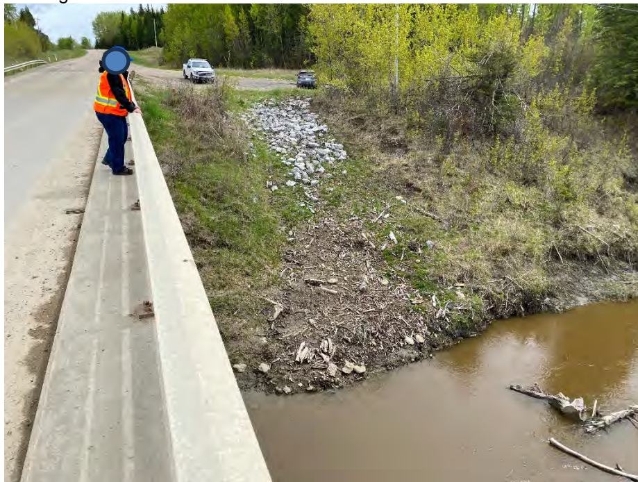
Photo 10: Riprap placed south of bridge along previous erosion channel. Driftwood collected near the east pier. Looking southeast.
