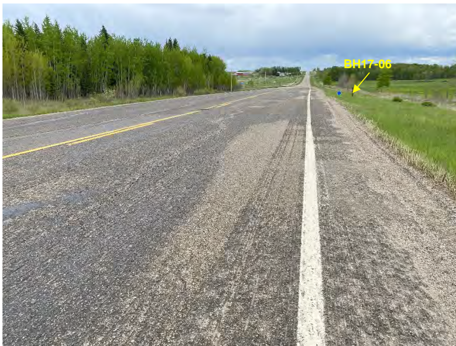
Photo 4: Pavement cracking on EBL. Looking east.
