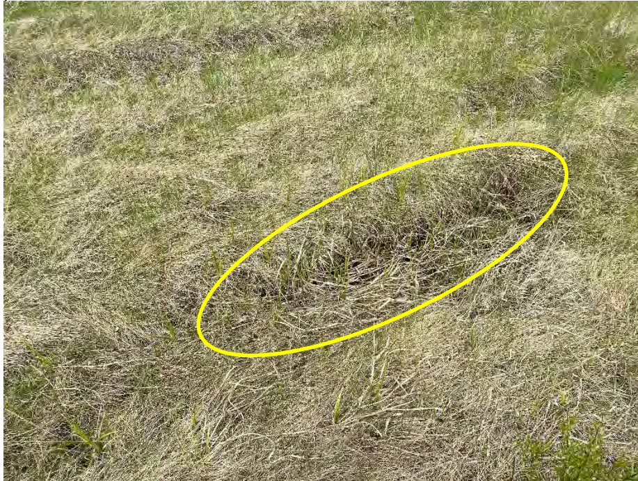
Photo 7: Depression in the north ditch near BH17-01. Looking north.
