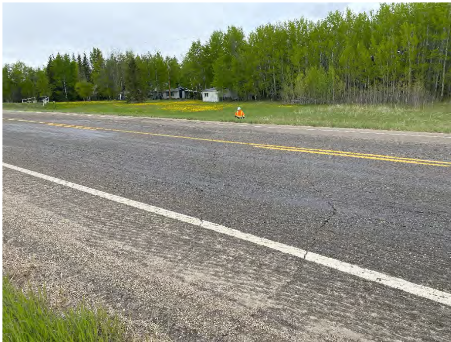
Photo 2: Diagonal cracking across milled pavement, looking northwest.
