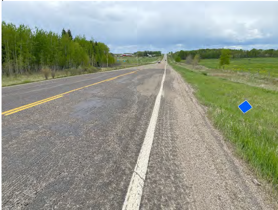
Photo 5: Pavement cracking on EBL. Looking east.
