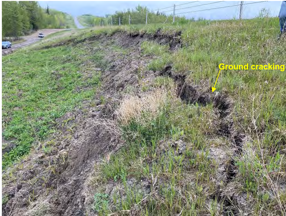
Photo 3: Backslope of failure and ground cracking to the south of the scarp. Looking northeast.
