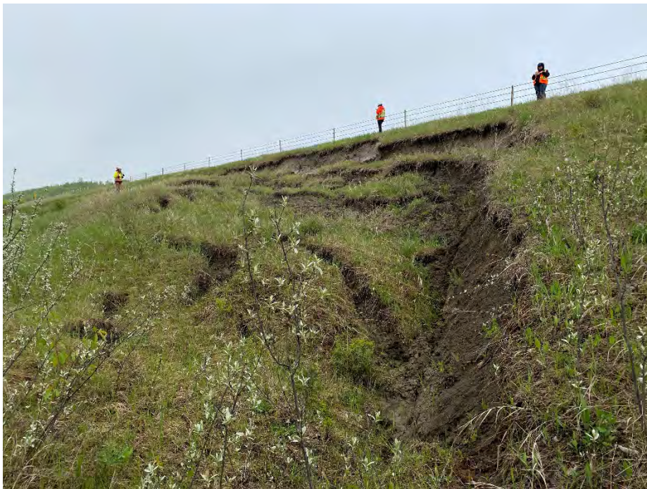
Photo 6: Slump on north end of east sideslope. Looking southwest from toe.
