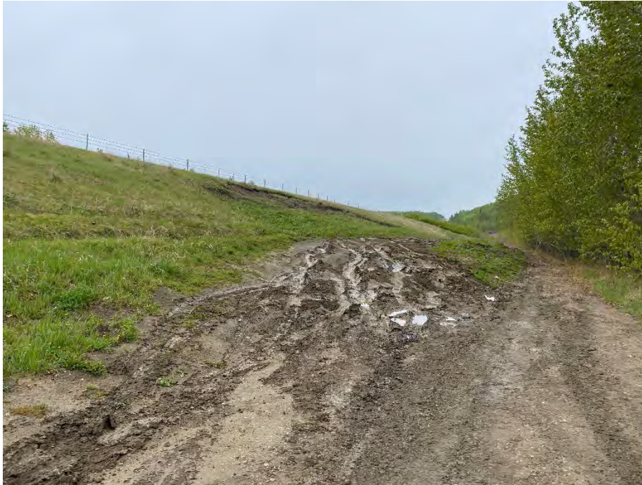
Photo 1: Failure at north extent of west side slope. Service road at landslide toe has been blocked. Looking south.
