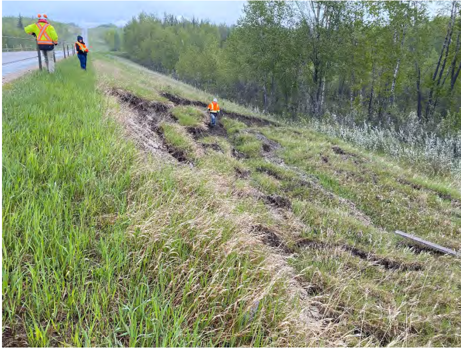
Photo 7: Northern slump on east sideslope. Looking northeast.
