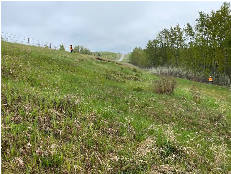
Photo 8: Middle slump on east sideslope. Looking north.
