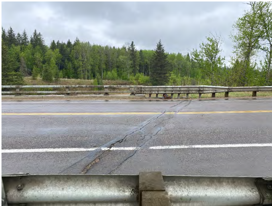
Photo 8: Pavement cracking at north abutment. Looking west.
