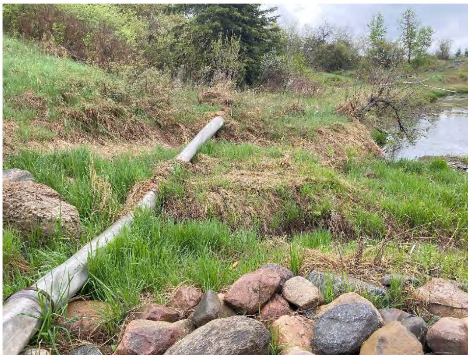
Photo 6: Undermined irrigation pipe along north bank, east of the bridge. Looking southeast.
