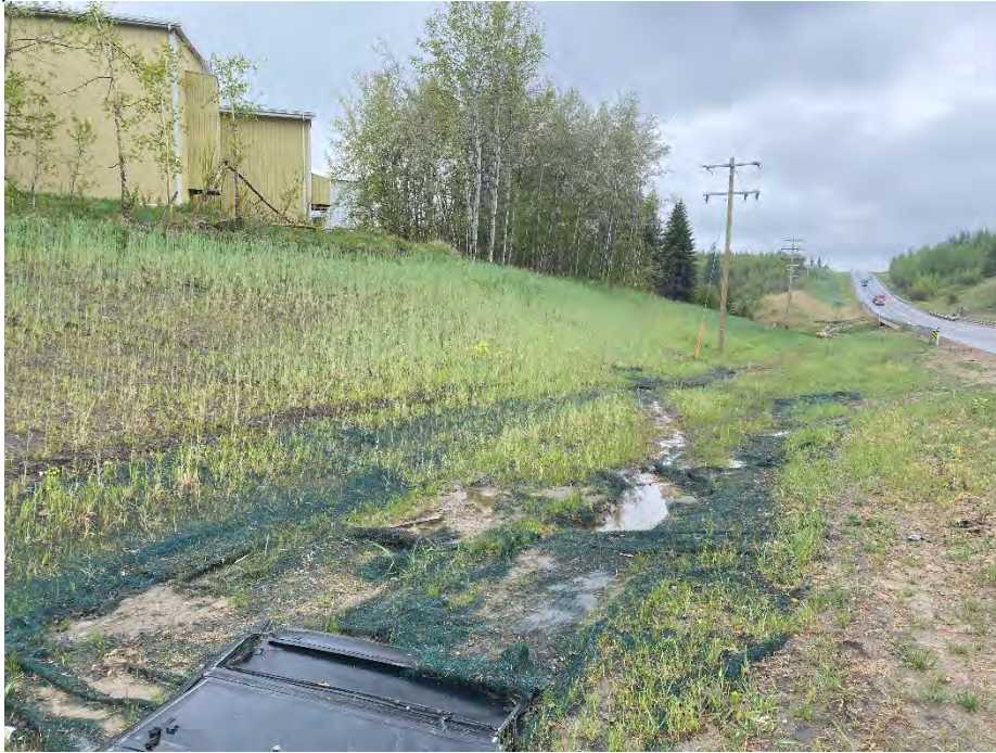
Photo 3: Erosion control blankets, debris and ponded water in east ditch, looking south.
