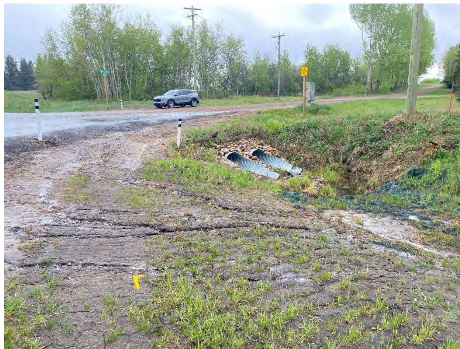
Photo 2: Repaired culvert outlets, with erosion channels off highway. Looking northeast.
