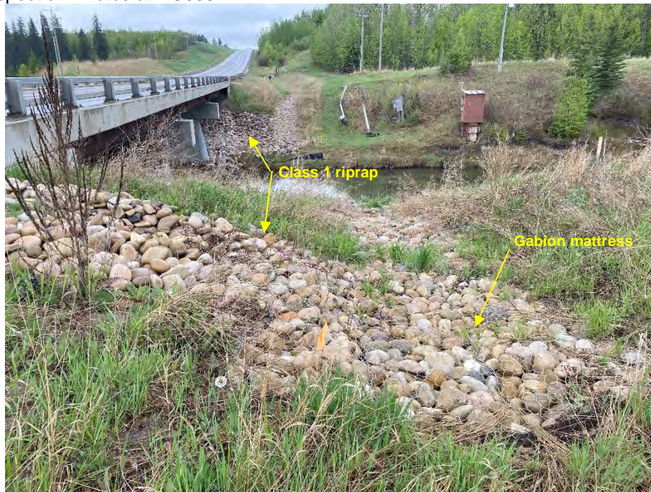
Photo 5: Remediation on west side of bridge, looking south.
