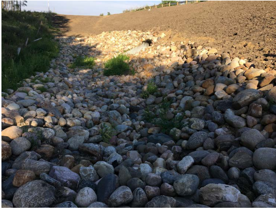
Photo 5 – Looking west across the freshly riprapped culvert outlet (July, 2017).
