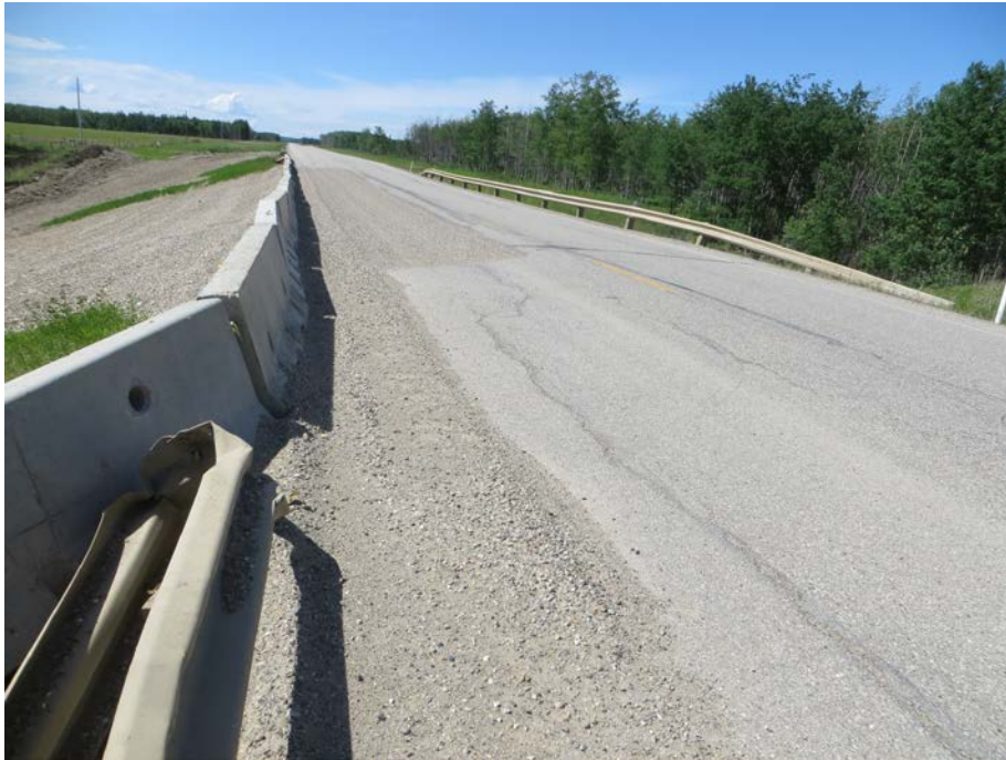
Photo 1 – Looking west along the highway over the repaired slide area.
