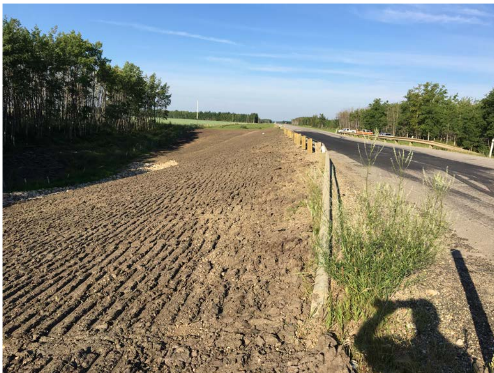
Photo 4 – Looking west along the repaired south hwy embankment (July, 2017).
