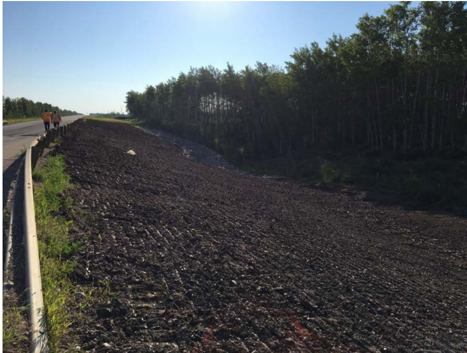
Photo 3 – Looking east along the repaired highway embankment (July, 2017).
