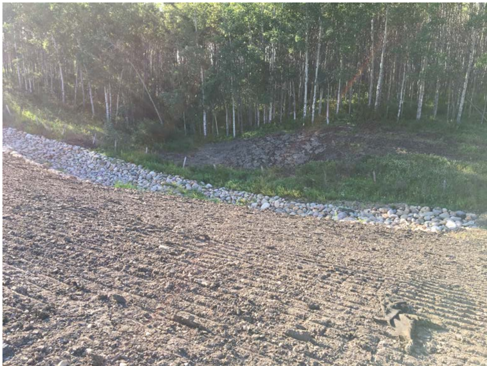
Photo 6 - Looking south over the new embankment and culvert outlet area (July, 2017).
