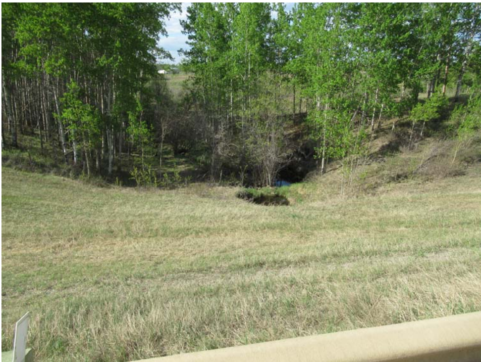
Photo 8 – Looking north across the downstream highway embankment and culvert outlet area.
