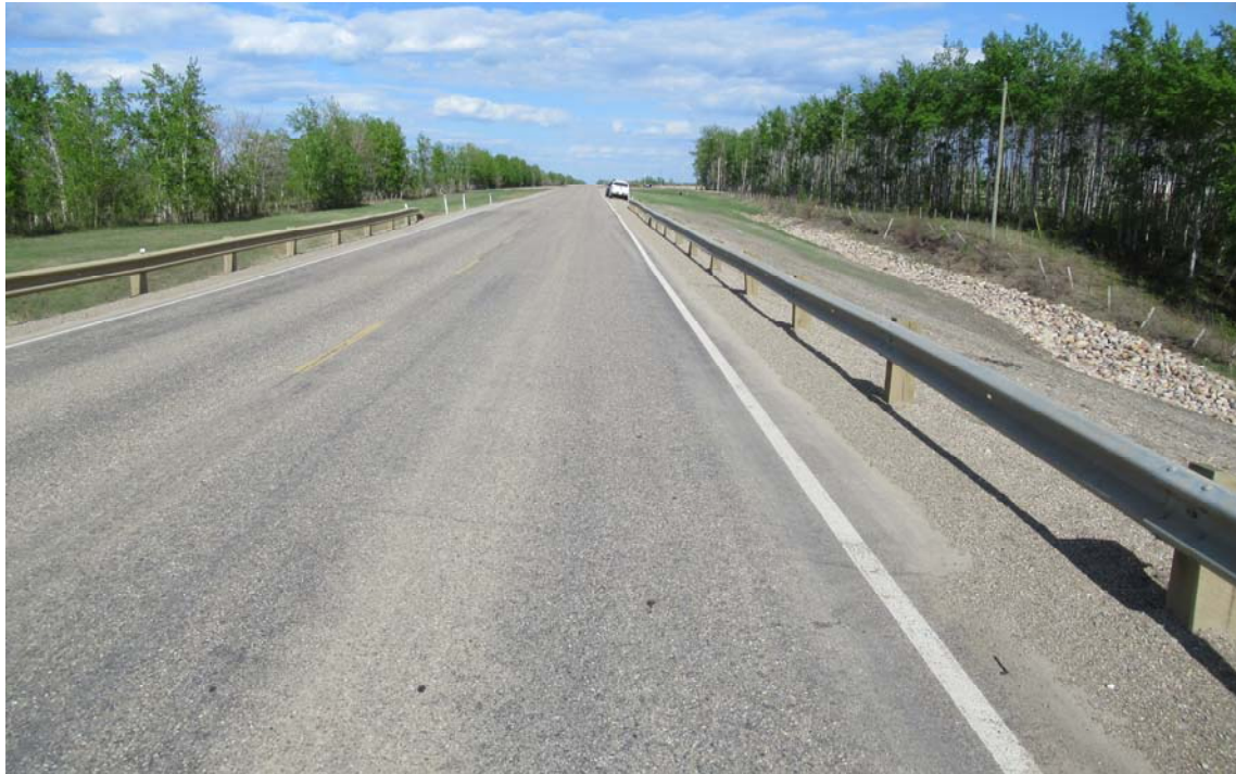
Photo 1 – Looking east along the highway over the repaired slide area.
