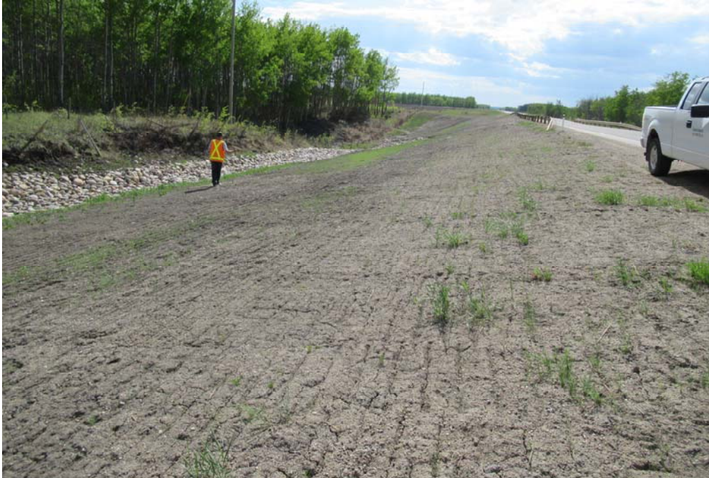
Photo 3 – Looking west along the south highway embankment from the east end.
