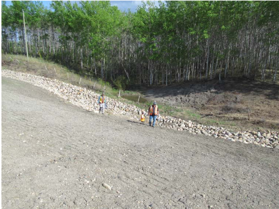
Photo 5 – Looking south over the new embankment and culvert inlet area.
