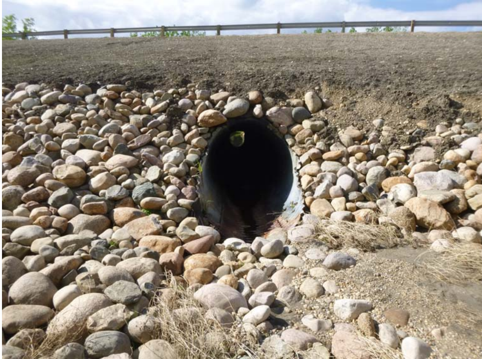
Photo 7 – Looking north through the culvert from the inlet area.
