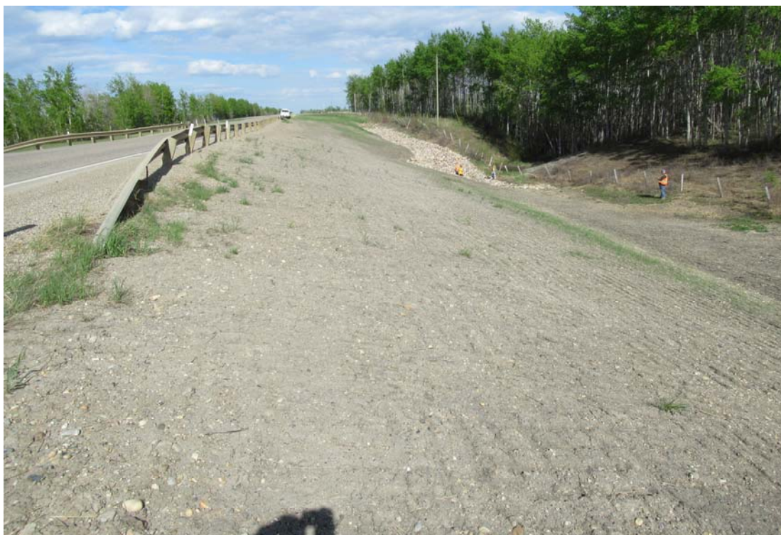
Photo 2 – Looking east along the repaired highway embankment.
