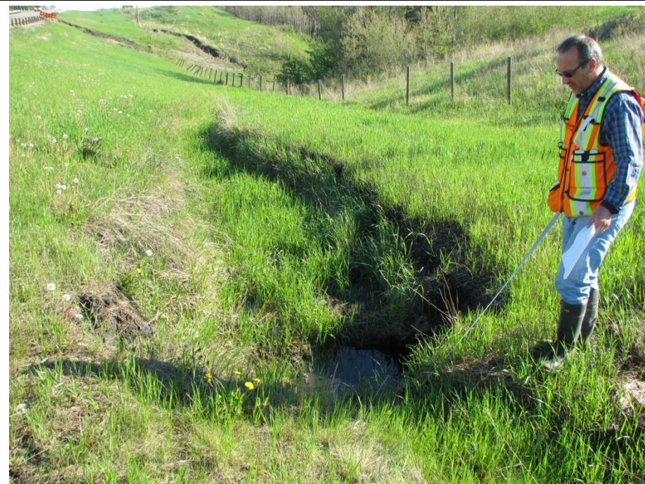
Photo 9. Looking northwards along the ditch in the SE corner of the site. Erosion gullies have slightly widened with sod falling into their base.
