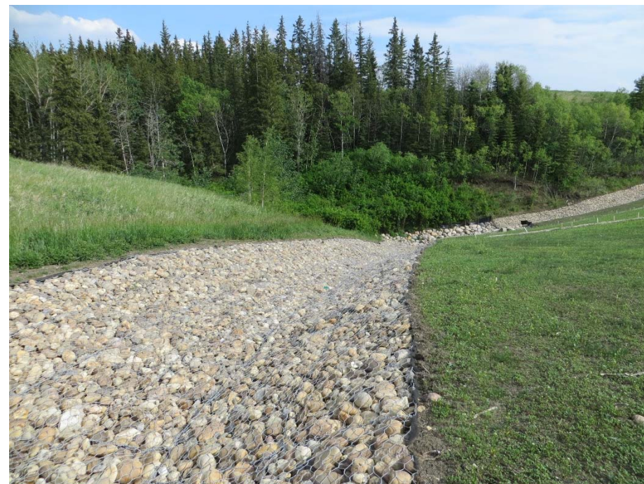
Photo 9. Looking southeast along gabion mattresses installed in northeast ditch in June 2014.
