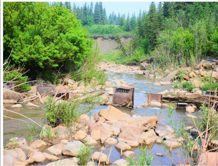
Photo 9. Pile weirs located in the streambed downstream of the bridge.
