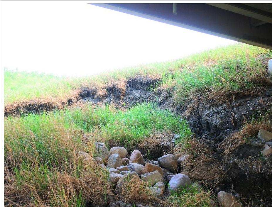
Photo 12. Looking southeast at the scarp and flank of Slide 2.
