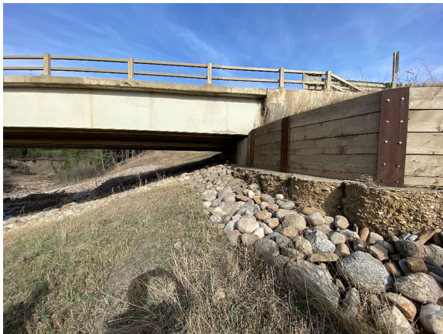
Photo 4. Looking east at the corner of the pile wall and settled riprap.
