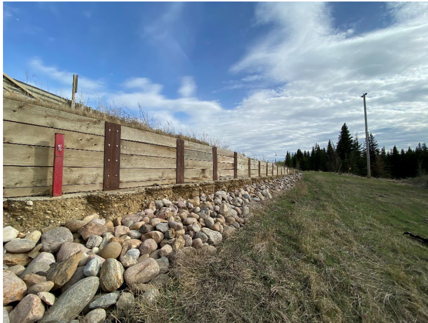
Photo 3. Looking southeast at riprap that appeared to have settled on the downslope side of the pile wall.
