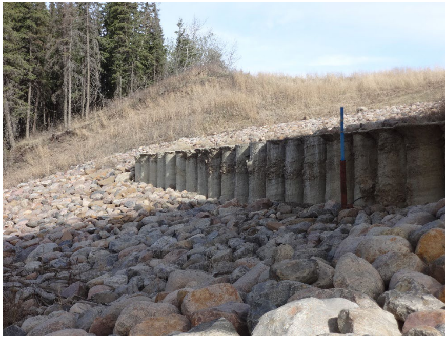
Photo 7. Looking southeast at riprap that settled below the east pile wall.
