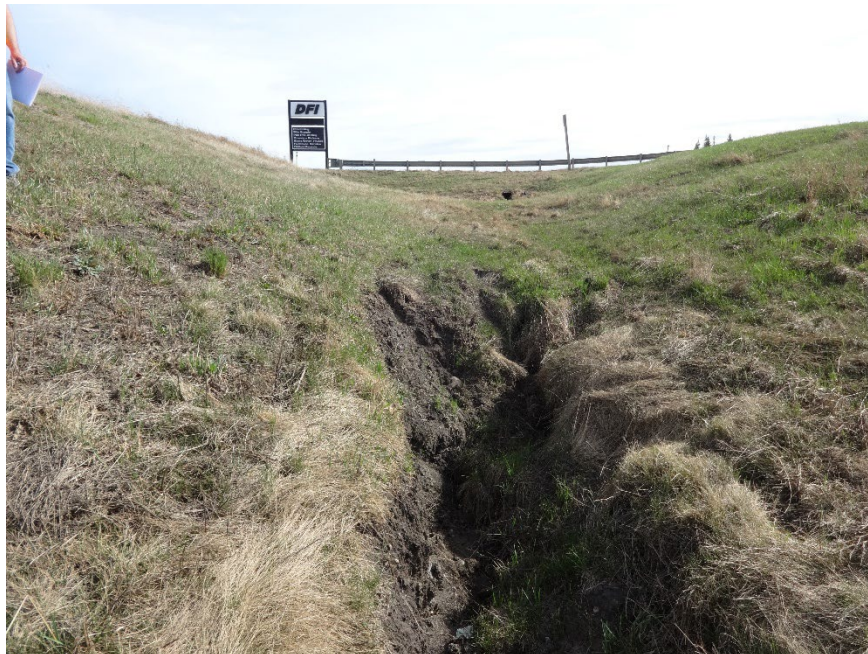
Photo 6. Looking south at erosion gully that has formed east of the south side of the bridge.
