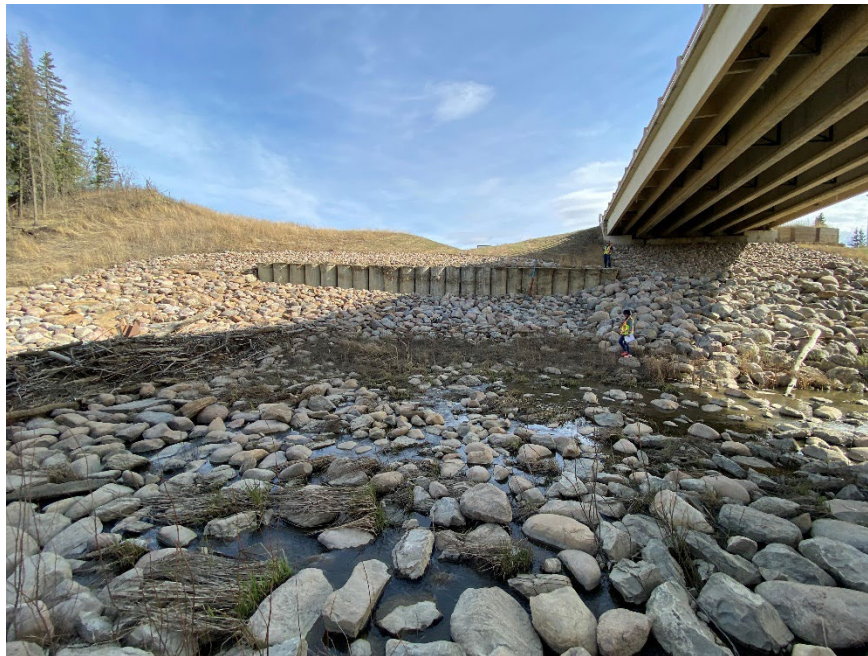
Photo 8. Looking south towards the east pile wall and riprap.
