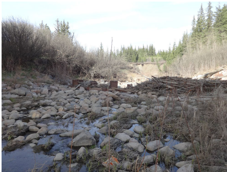
Photo 10. Looking northeast at debris that has accumulated in the pile weirs.
