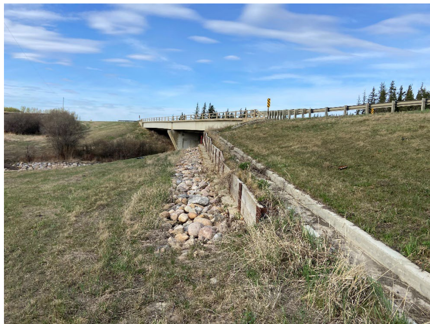
Photo 2. Looking northeast at the concrete drain trough above the west pile wall.
