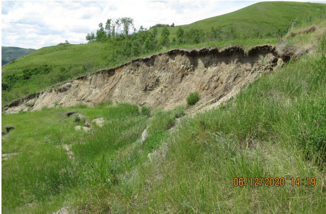
Photo 9: Looking west along the backscarp
