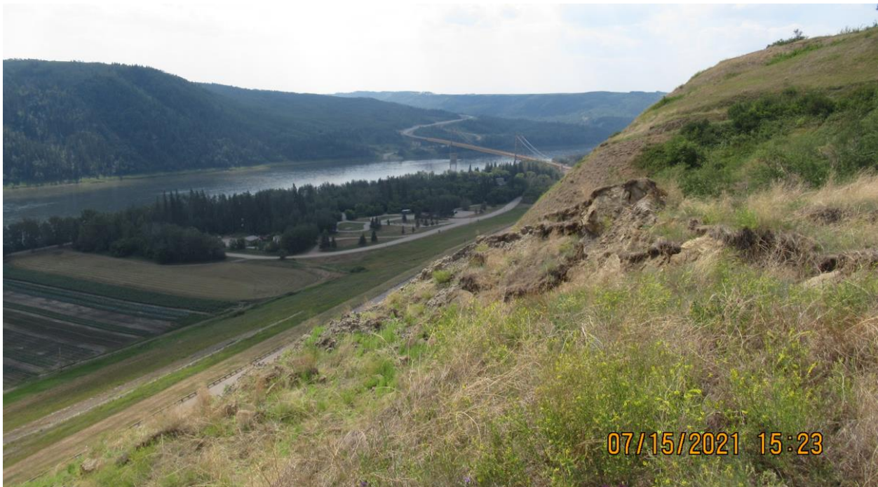
Photo 10: Looking west along the toe of the slide
