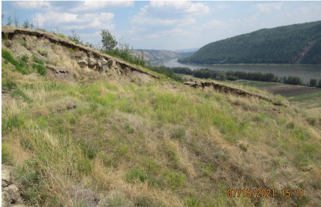
Photo 7: Looking east from landslide backscarp
