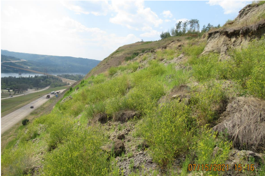
Photo 11: Looking southwest within the landside mass; note active toe roll
