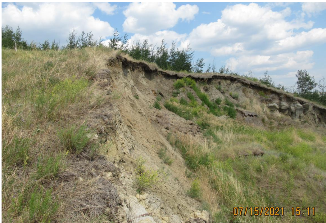
Photo 6: Looking northeast along backscarp of the landslide
