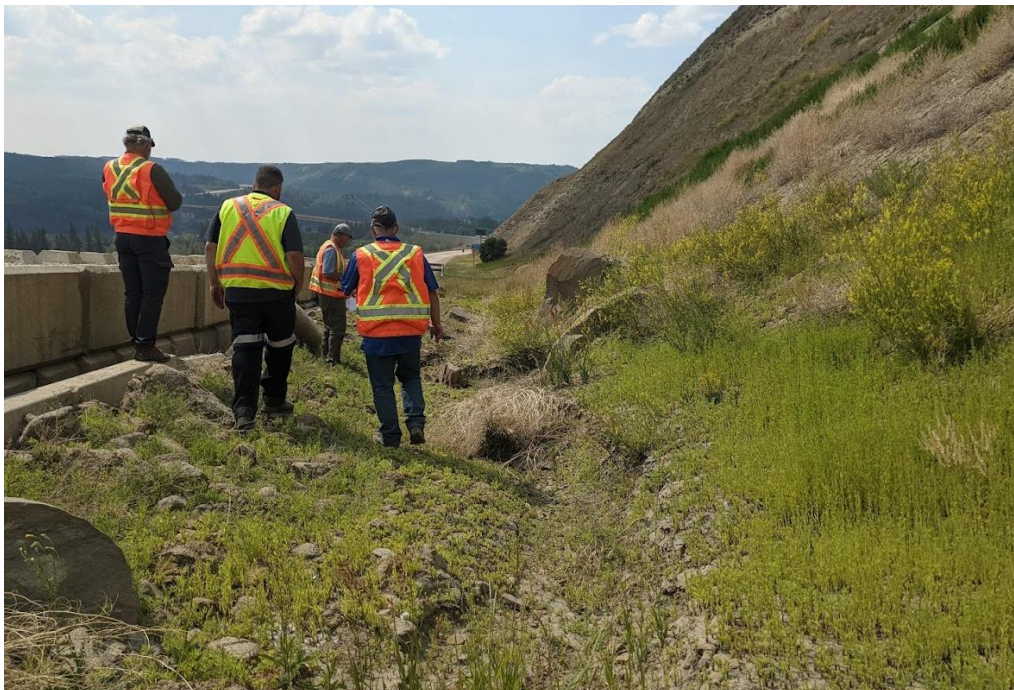
Photo 4: Looking west at the accumulated sandstone slabs, talus, boulders, and soil chunks appears to be approximately the same as 2020. But, with some vegetation growing
