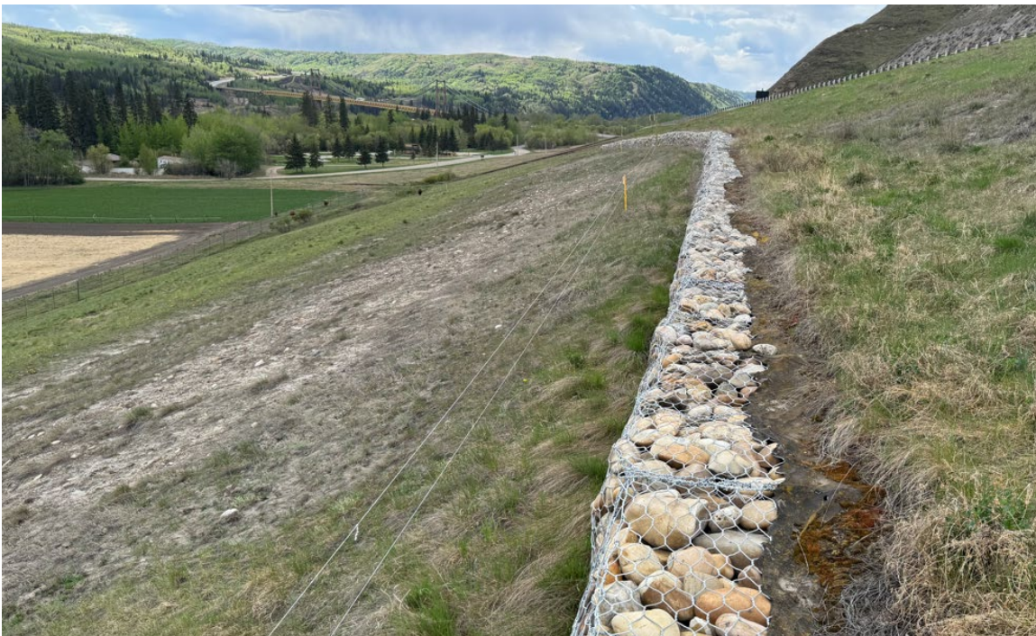
Photo 10: Gabion Basket. Acceptable condition in 2024
