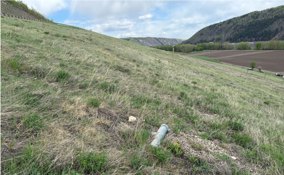
Photo 9: Subdrain outlet located upslope from gabion basket. Dry in 2025
