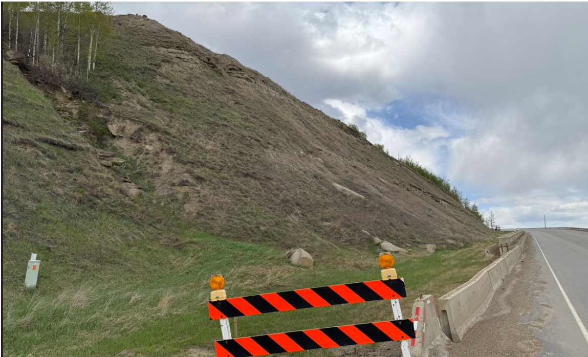
Photo 8: Looking east at steep rock backslope and a few sandstone blocks accumulating behind the Concrete Jersey Barrier
