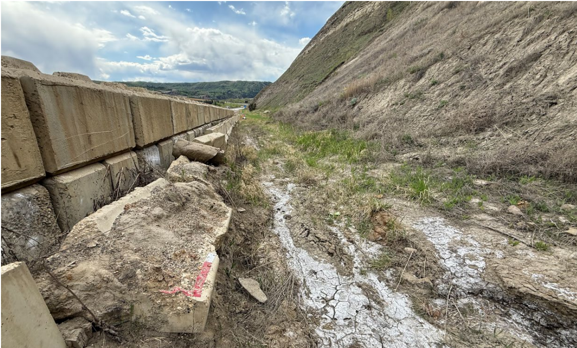
Photo 4: Area where sandstone slabs, talus, boulders accumulated the most prior to the 2022 clean up. Note fresh slumping on the lower backslope on the right of the photo. Concrete blocks that are in contact with landslide debris are starting to disintegrate.
