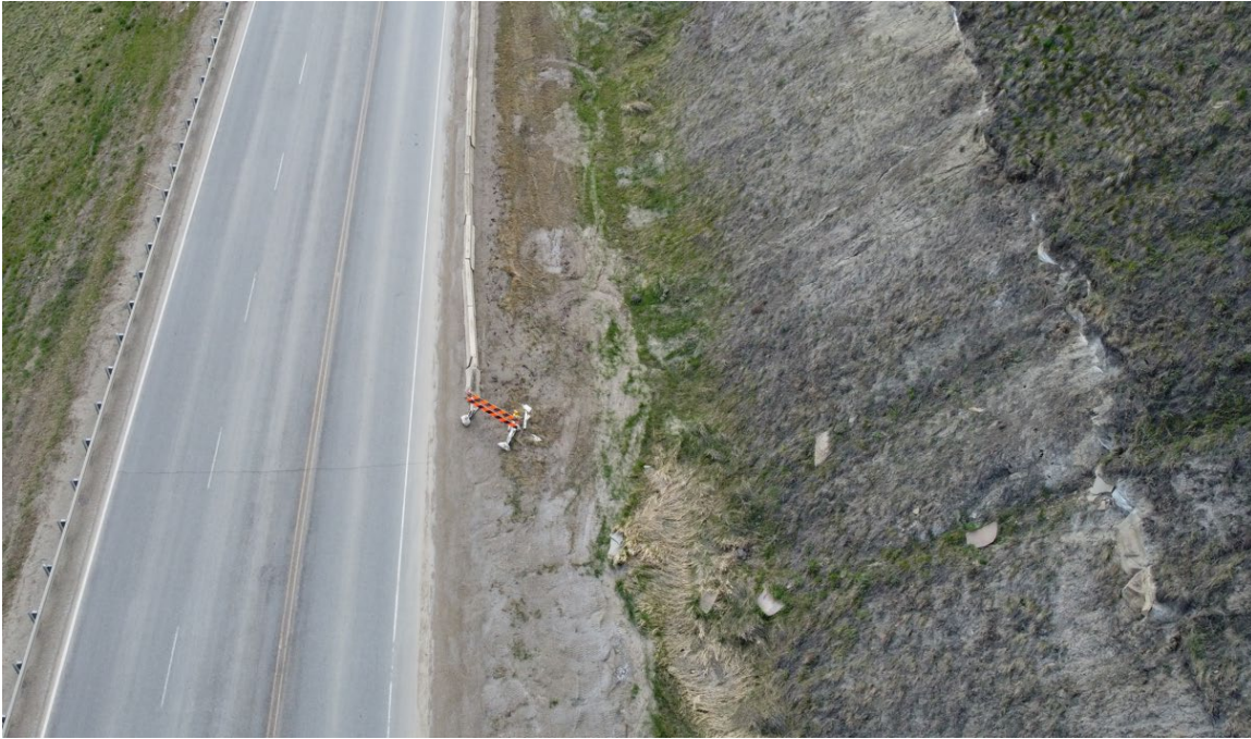
Photo 11: Lower sandstone ledge starting to crumble 20 m east of Jersey barrier.
