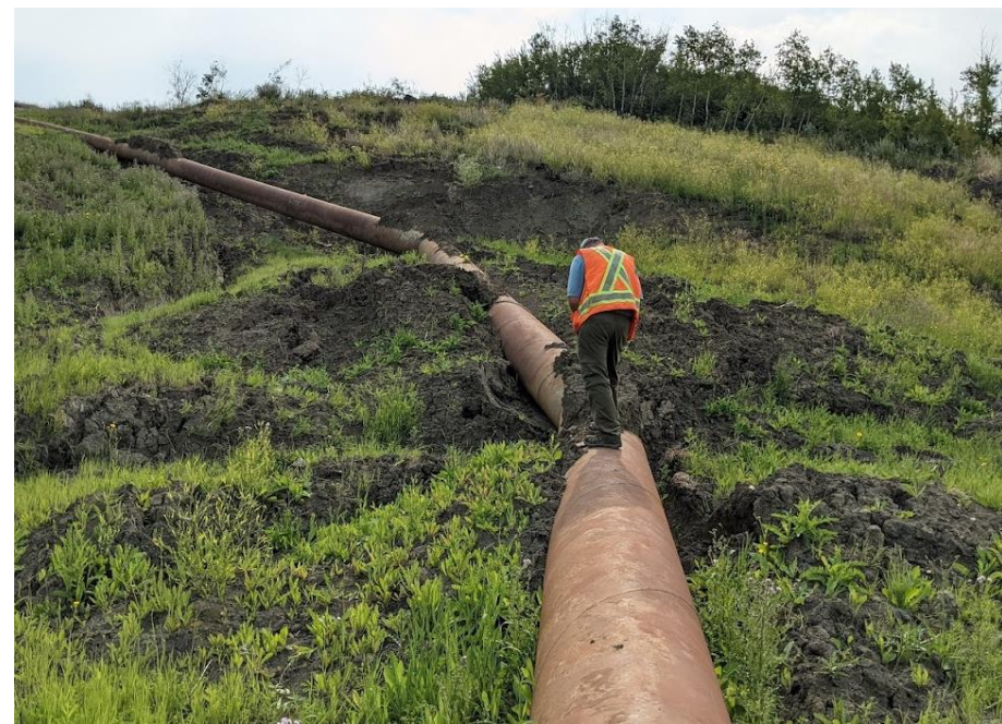
Photo 7. Looking upstream at SWSP middle bend and soil berm.
