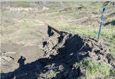
Photo 2. Looking west from the crest of the valley bench. Note seepage on the bottom left of the photo
