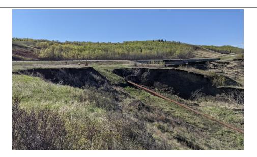
Photo 3. Looking south from 2+200, about 110m west of Hwy 2:68. Overall increase in slide activity along the backscarp in the upper portion of the Elephant Trunk drainpipe since 2021. Note up to 1.3 m of settlement of slide mass under the **SWSP** downslope of where it exits the fill cover.
