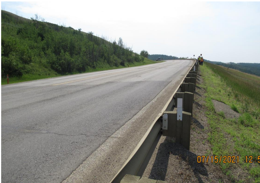
Photo 7. Looking from the shoulder of the SBL at Sta. 1+660 across the dip in the highway at the north end of the 1+800 slide.
