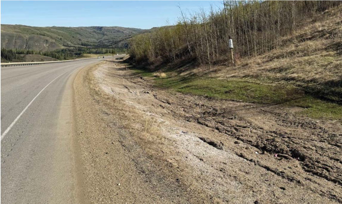
Photo 5: Looking north from Sta. 1+800. The erosion gully noted on the ditch up to 1.7 m wide and 0.7 m deep in 2024 was regraded. Currently rills are less than 200 mm wide by 200 mm deep.
