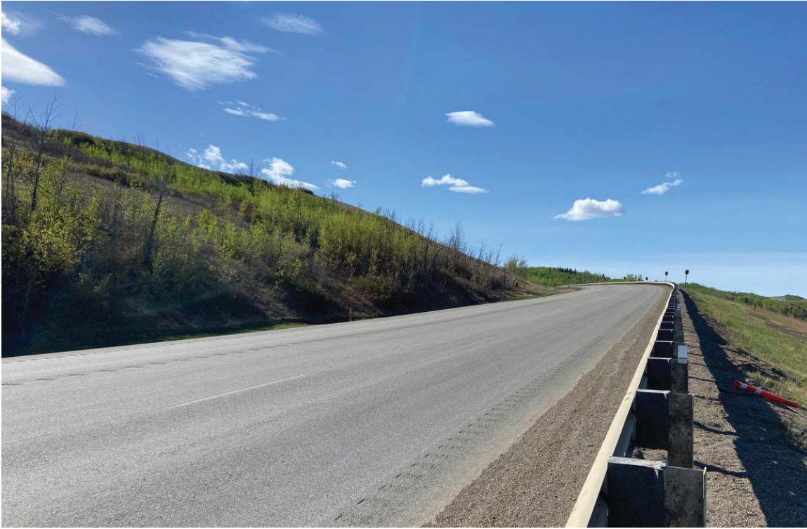
Photo 7: Looking south at the north end of the 1+800 slide. No slide cracks or dips visible on the recently (2024) paved highway surface.
