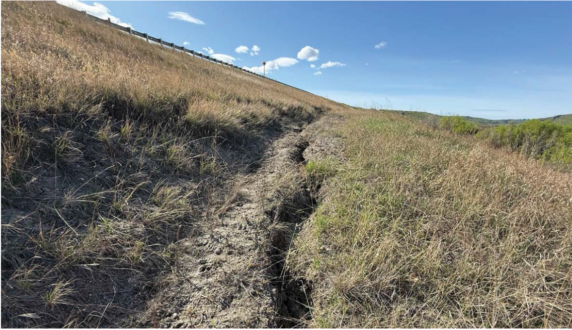
Photo 15: Looking south at slumping occurring from Sta. 1+480. Scarp measured 1.3 m deep in 2025
