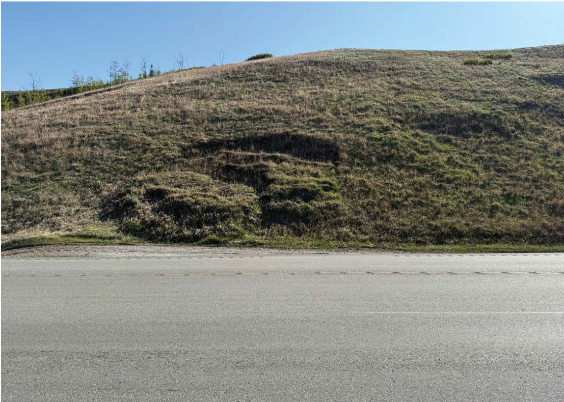
Photo 3: Looking east at backslope skin failure at Sta. 1+950. More active in 2025
