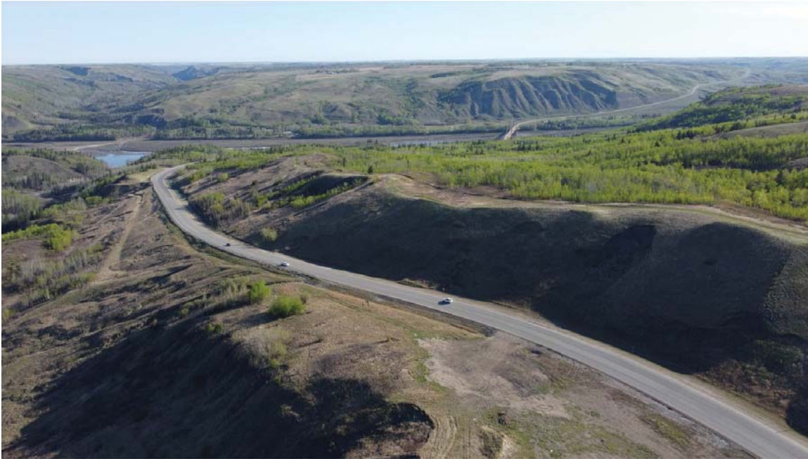
Photo 17: Drone view showing slumps along the highway sideslope and backslope. Overall backslope slumps are more active and partially blocking the upslope ditch.
