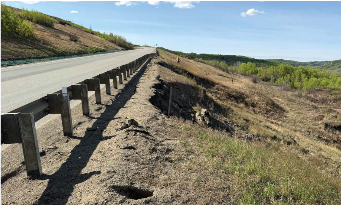
Photo 13: Looking south from Sta. 1+390 at the backscarp of the 1+400 slide.
