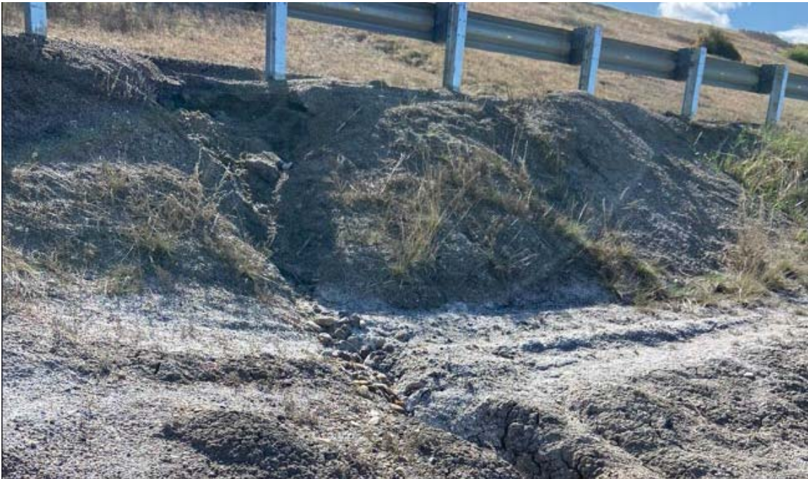
Photo 9: Looking north near Sta. 1+550 at erosion rills and gullies on the highway side slope becoming worse.
