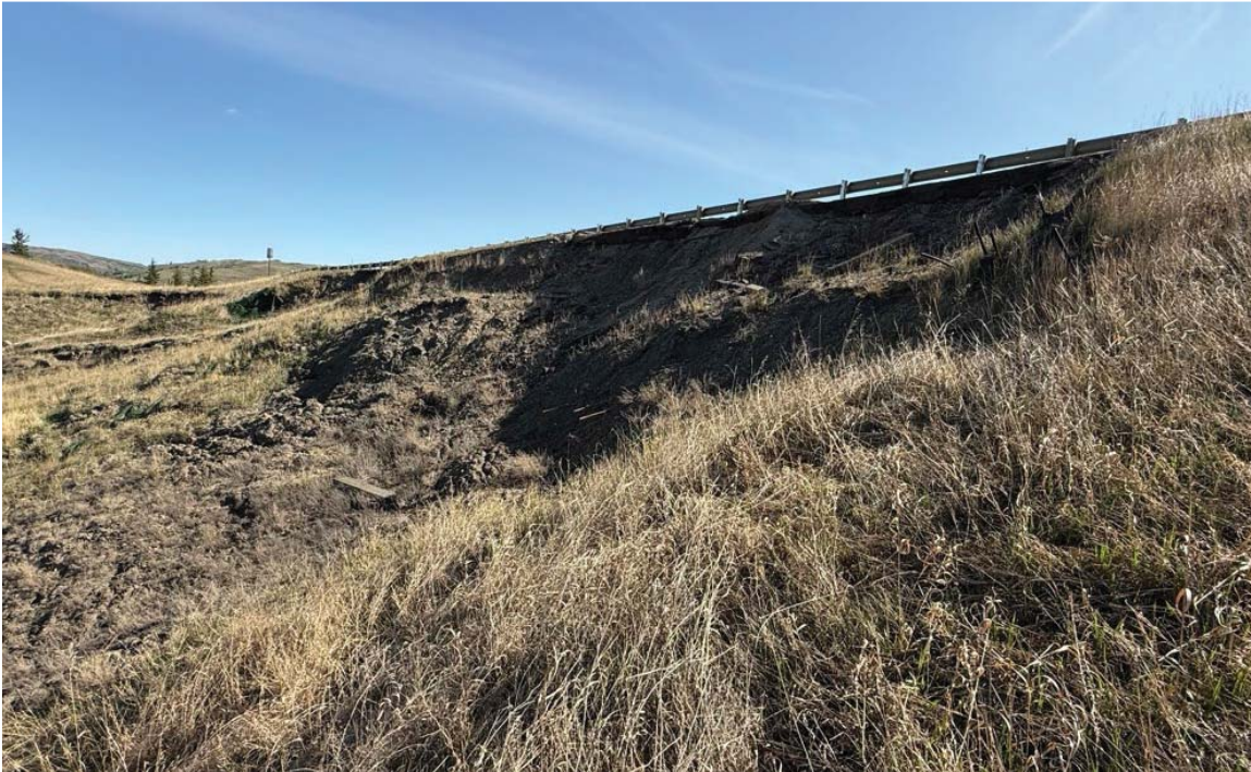
Photo 11: Looking east at failed soil matting and soil nails which were installed in August 2010 at Sta. 1+450 slide. Backscarp (5 m to 7.5 m high) continues retrogressing and impacting the highway embankment.
