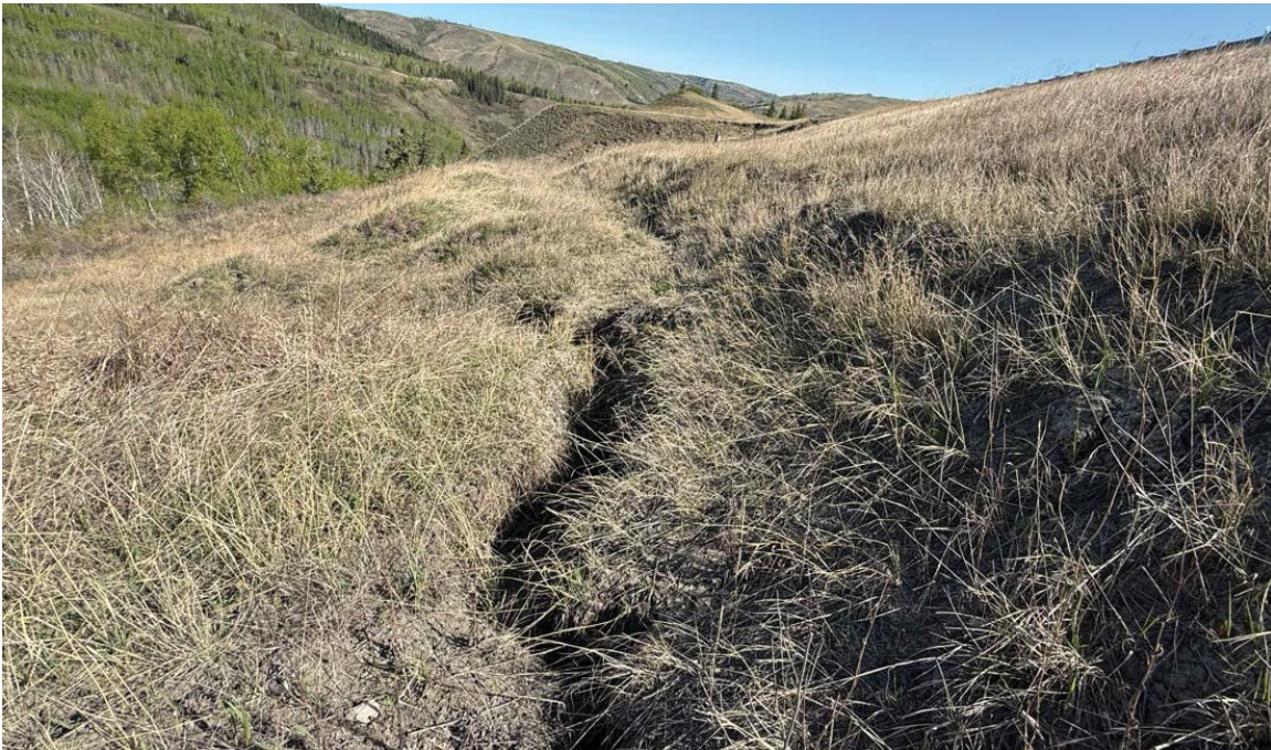
Photo 16: Looking north at slumping occurring from Sta. 1+500..
