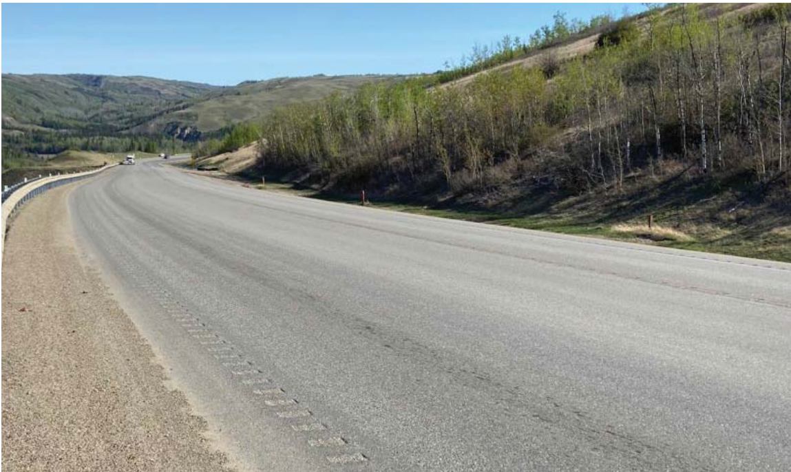
Photo 6: Looking north across the former dip in the highway at the south end of the 1+800 slide. No slide cracks or dips visible in the recently (2024) paved highway surface.
