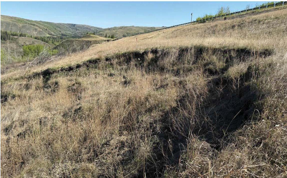
Photo 8: Looking north near Sta. 1+670 at slumping occurring on the highway side slope approximately 20 m from the edge of pavement. More movement noted in 2025
