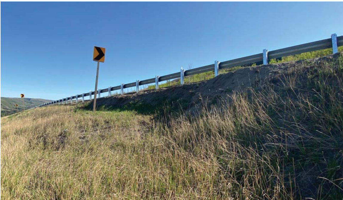
Photo 4: Looking north from Sta. 1+890 at the slump in the sideslope of the SBL. More movement in 2025. The scarp is 1.8 m high and 1.0 m from the guardrail.
