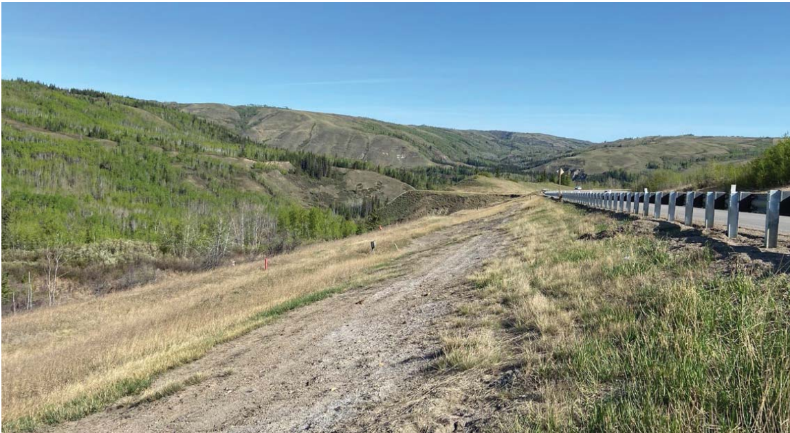
Photo 10: Looking north near Sta. 1+560 at rough area (drill access bench) with some seepage and tension cracks. Access bench was damp in 2025
