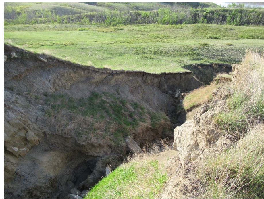
Photo 12. Looking southeast along the centerline culvert scour channel at mid-slope.
