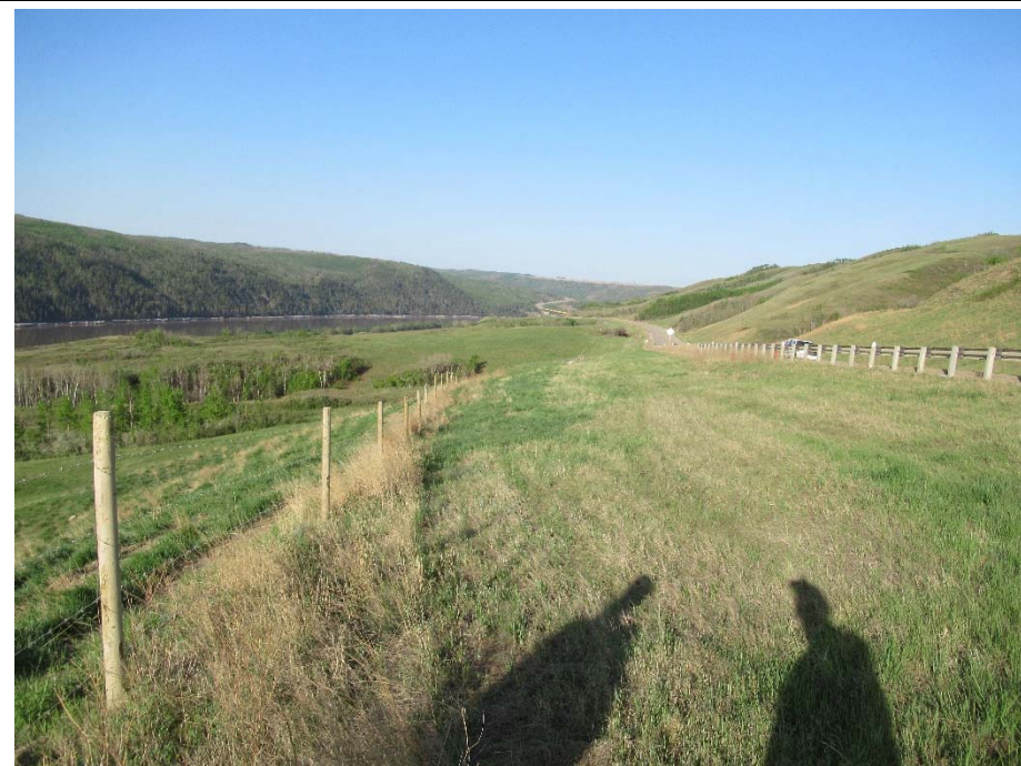
Photo 4. Looking southwest along the new pile wall built in 2015/2016. The pile wall is buried below ground. The grass catch in the area seeded in the highway sideslope at the wall location is good. The bow in the new fence installed in 2016 is more pronounced than in 2017.
