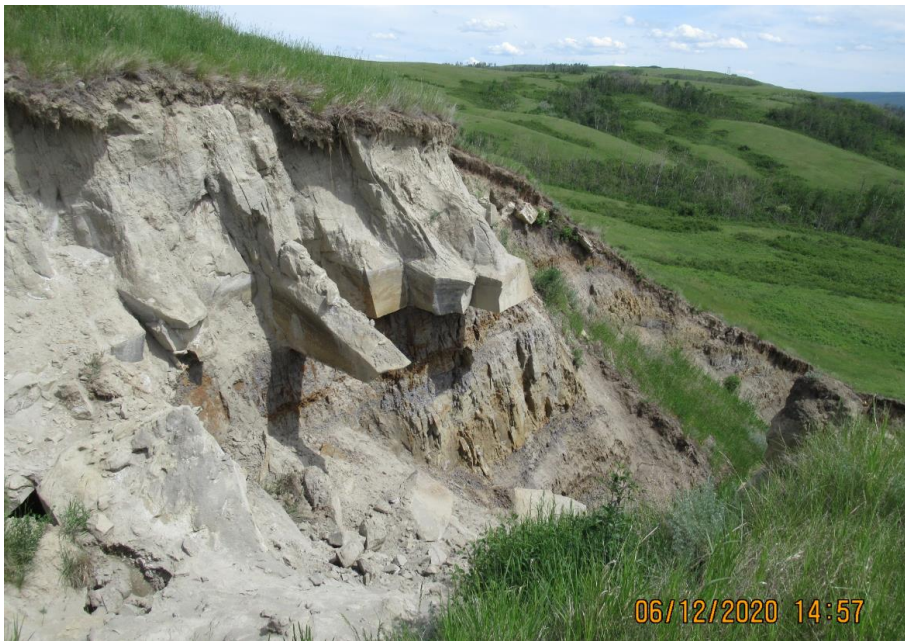
Photo 9. Looking north from the west side of the scour channel that is situated below the outlet of the centerline culvert.
