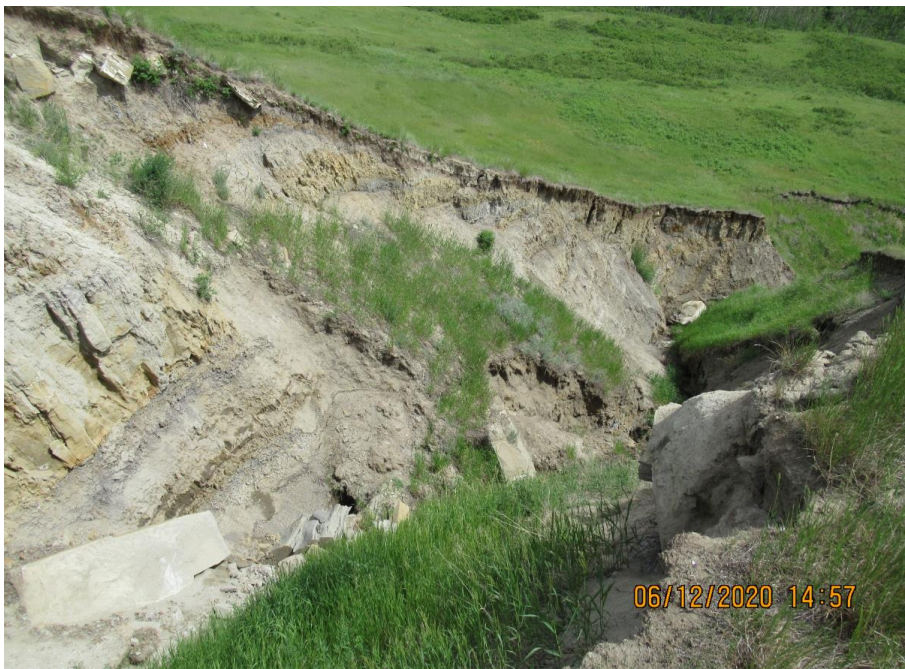
Photo 10. Looking southeast along the centerline culvert scour channel at mid-slope.
