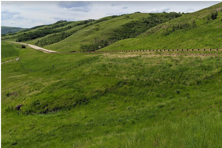
Photo 4. Looking southwest at landslide mass. Note the soil dropped up to 1.5 m below the pile wall and is now exposing the upper 0.5 m of the pile wall at the crest of the slide near the guardrail. The toe bulge is still well-defined at the bottom. The barbed wire fence is still being impacted by landslide movement. But, has not been broken yet.
