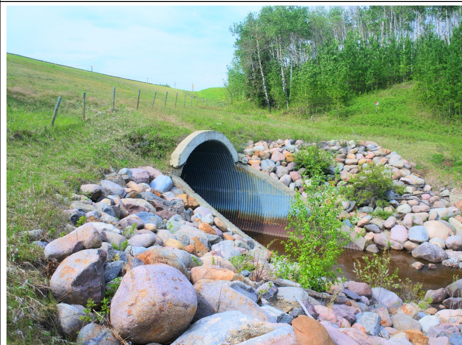
Photo 10. Looking northwest towards the 6.1 m diameter SPCSP centerline culvert.
