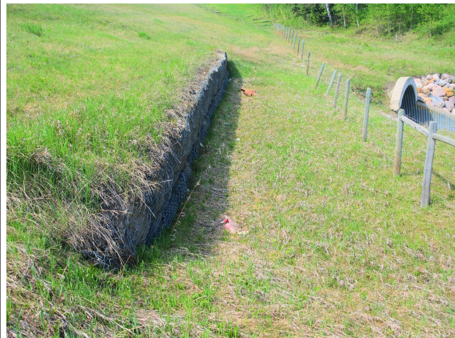
Photo 8. Looking northwest at gabion wall above CSP culvert outlet.
