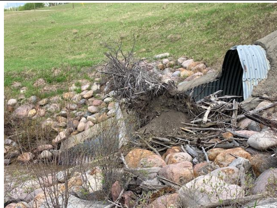
Photo 10. Looking northwest towards the 6.1 m diameter SPCSP centerline culvert inlet.
