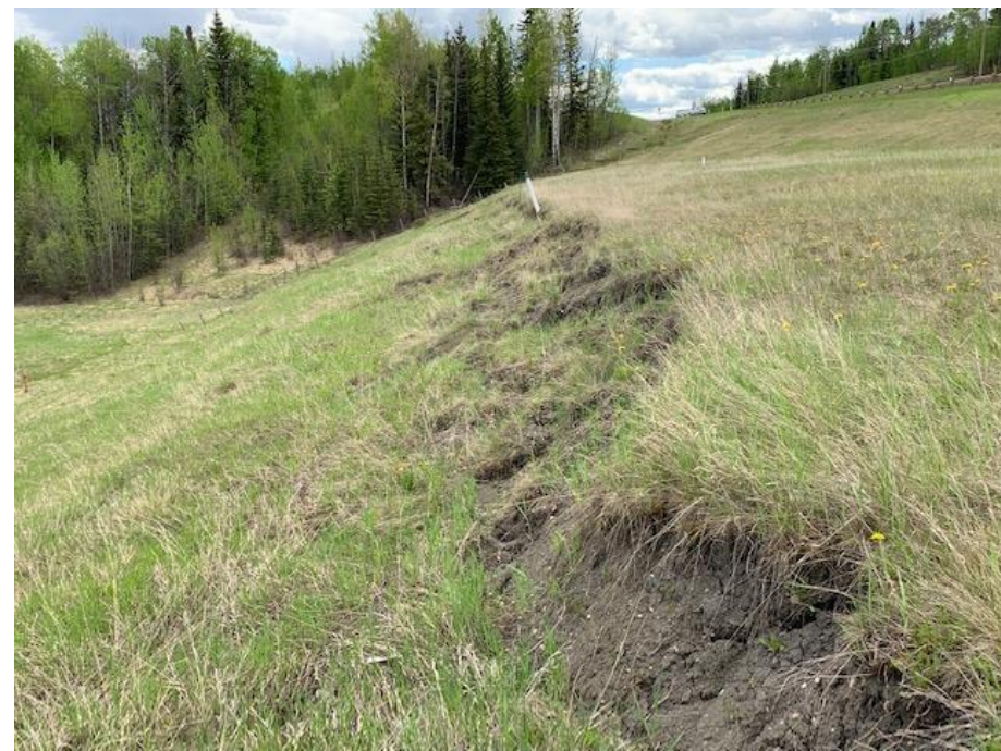
Photo 8. Looking southeast at relatively fresh slumping from head scarp.
