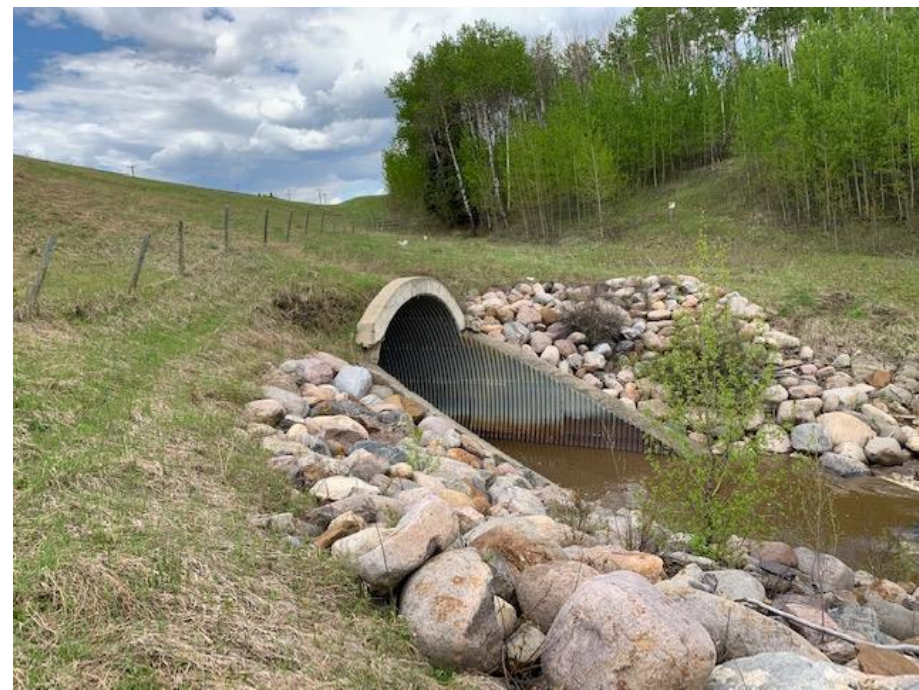
Photo 9. Looking northwest towards the 6.1 m diameter SPCSP centerline culvert outlet.
