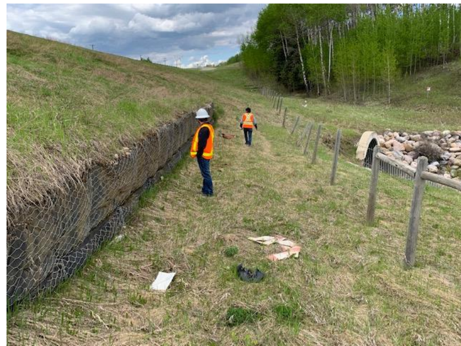
Photo 7. Looking northwest at gabion wall above CSP culvert outlet.
