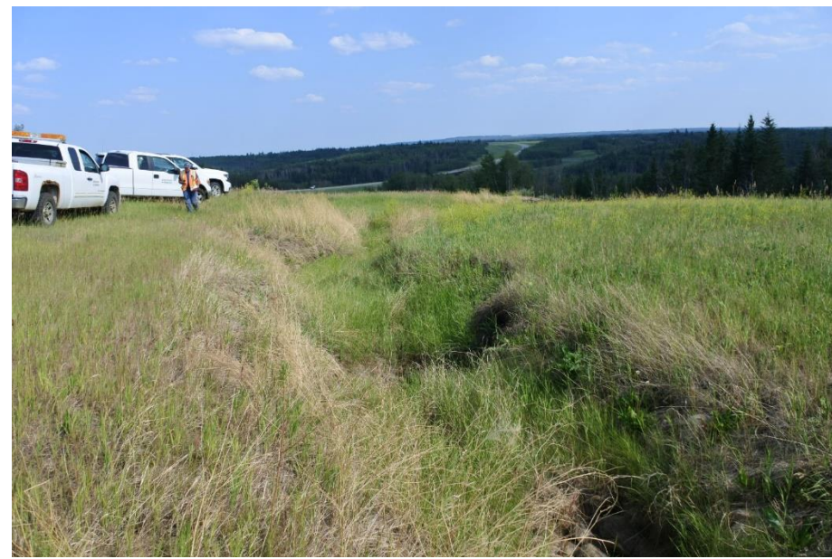
Photo 1. Looking south at erosion gully that has formed in the south ditch which was dry due to warm weather in 2021.
