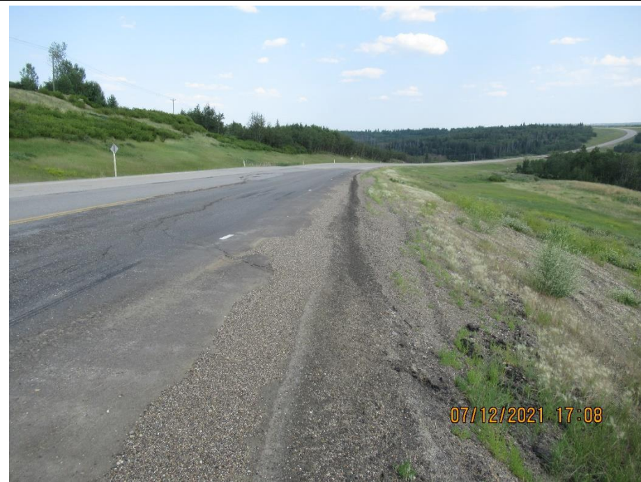
Photo 6. Looking east from the shoulder of the EBL of Hwy 49:06 at the westmost dip in the fall 2020 ACP patch. Note the scarp within the embankment
