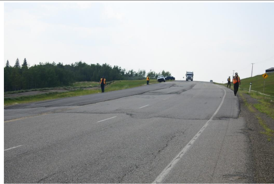
Photo 10. Looking northwest from the EBL of Hwy 49:06 at the south end of the site.
