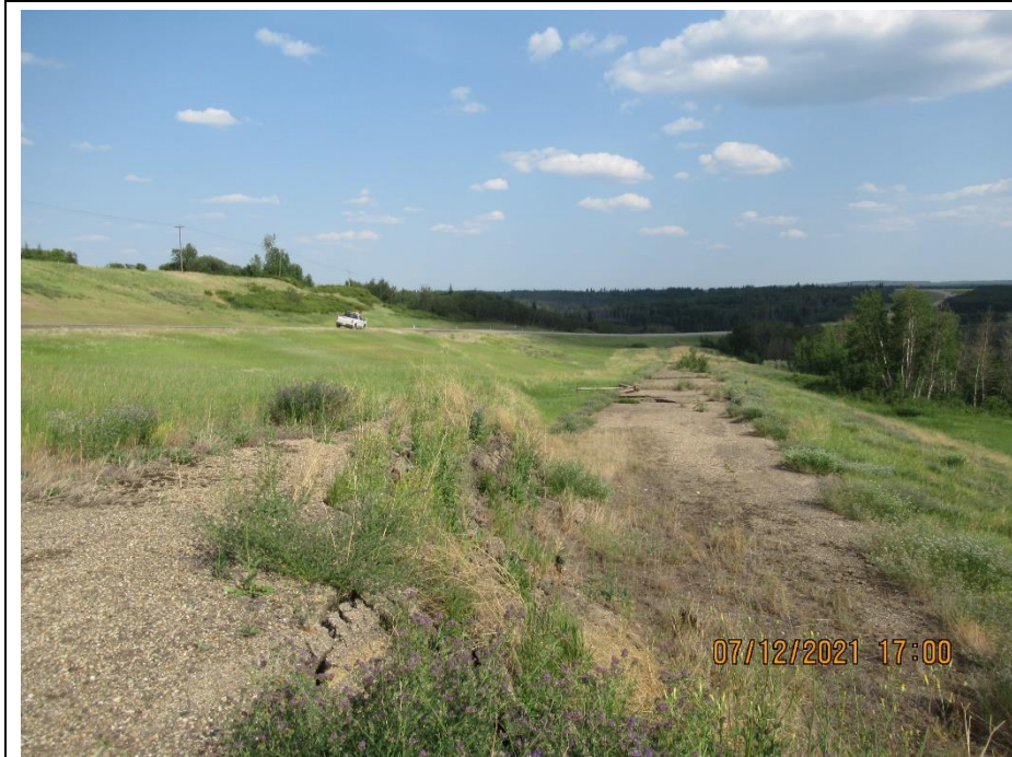
Photo 3. Looking southeast at where scarp crosses the old highway alignment.
