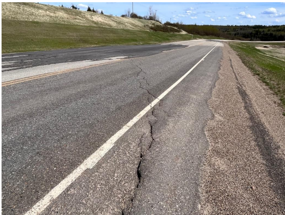
Photo 12. Looking southeast at the northwest end of the site at scarp crack open on the SBL shoulder.
