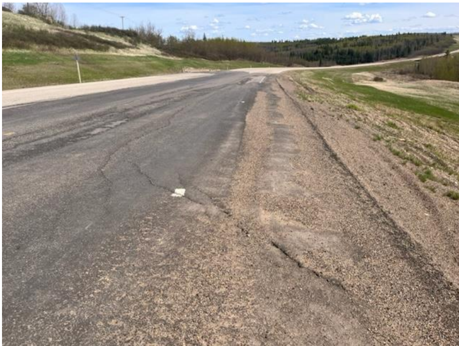
Photo 6. Looking east from the shoulder of the EBL of Hwy 49:06 at the westmost dip in the 2021 ACP patch.
