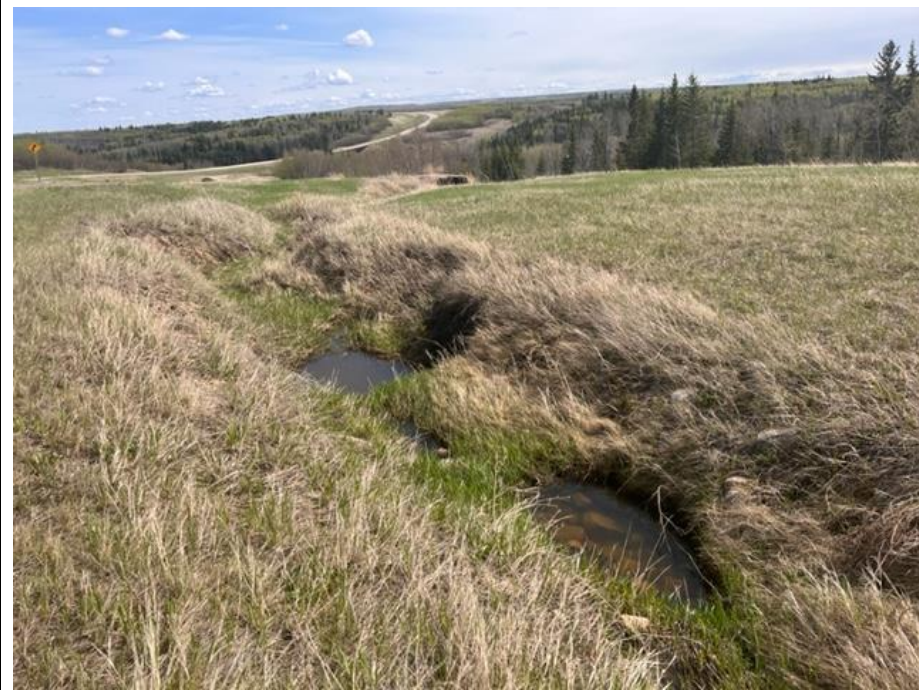
Photo 1. Looking southeast at erosion gully that has formed in the south ditch which had pooling water in it in 2022.
