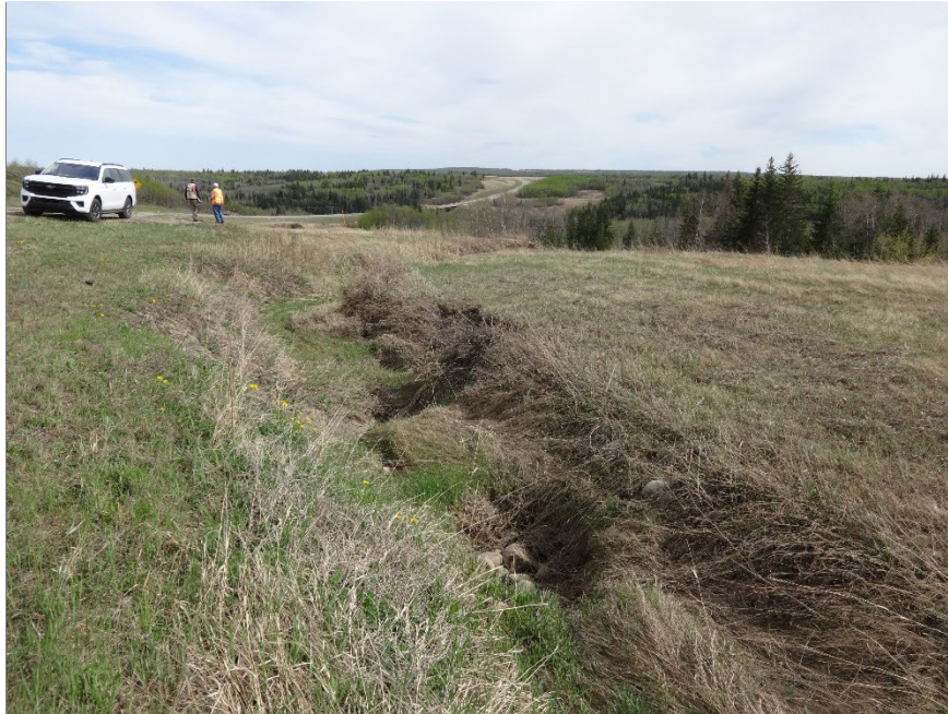
Photo 1. Looking southeast at erosion gully that had formed in the south ditch that had pooling water in it in 2022 but the scour holes were mainly dry with slight moisture in 2025.
