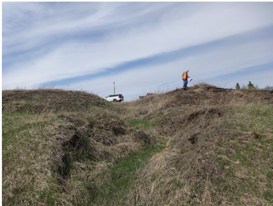
Photo 2. Looking north from edge of erosion gully. Note the ditch along south side of highway tails off and has been the contributor to this erosion.
