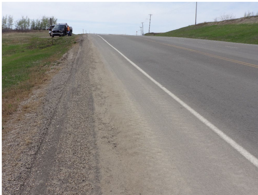
Photo 12. Looking northwest at the ACP overlay placed at the site.
