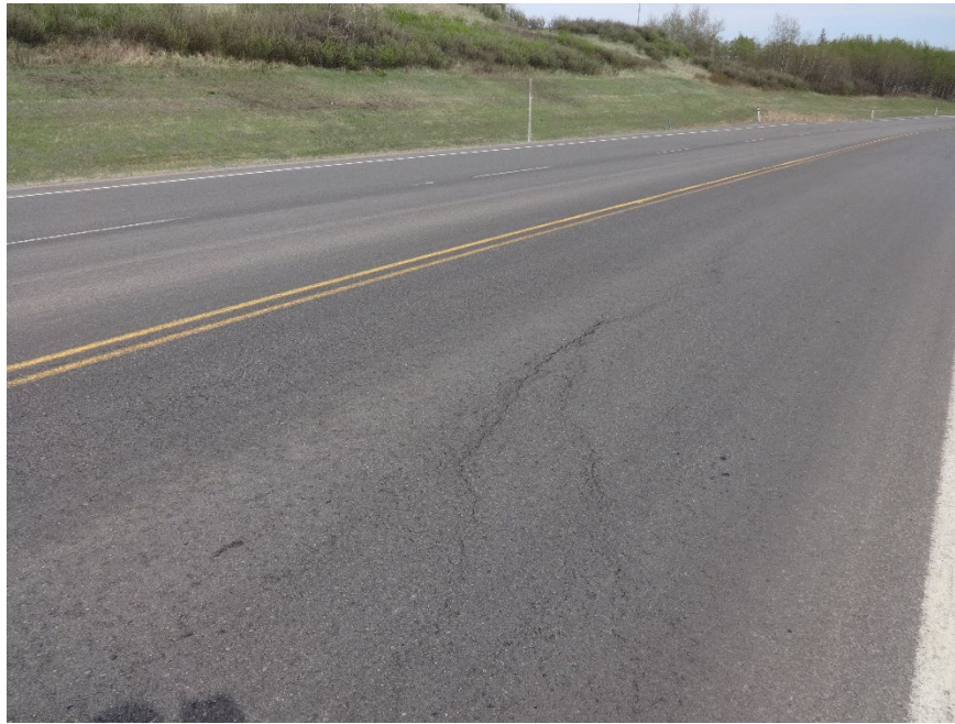
Photo 9. Looking east from near the middle of the site where crack is showing in EBL.
