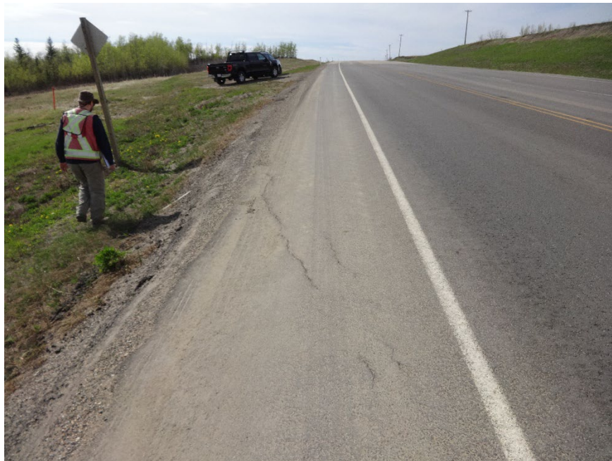
Photo 14. Looking northwest at hairline cracks showing in the eastbound lane shoulder at the northwest extent of the site.
