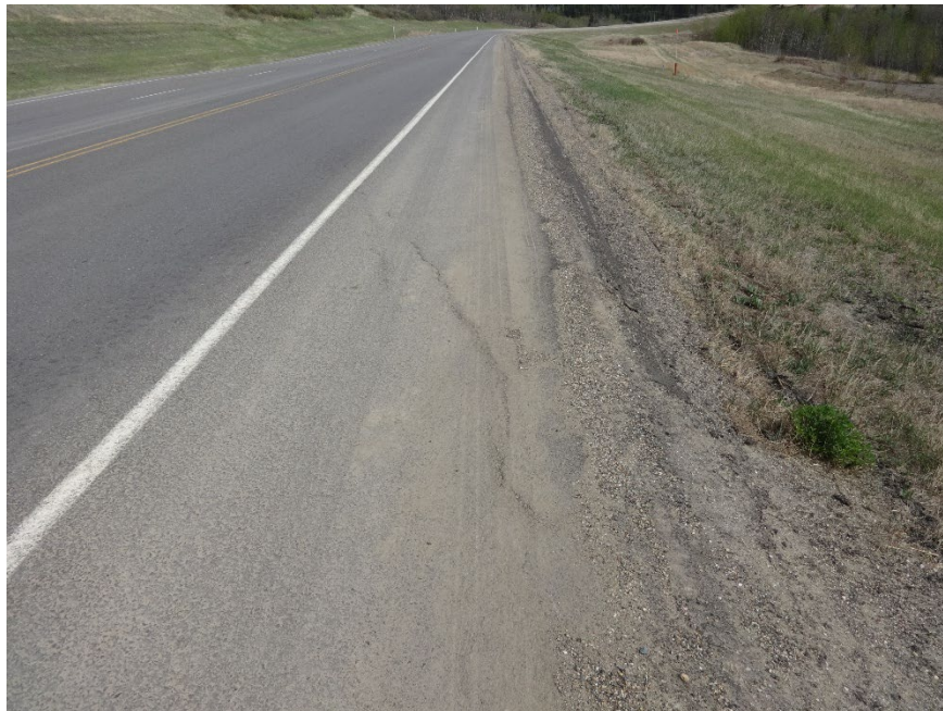
Photo 6. Looking east from the shoulder of the EBL of Hwy 49:06 at the hairline cracks in the shoulder.
