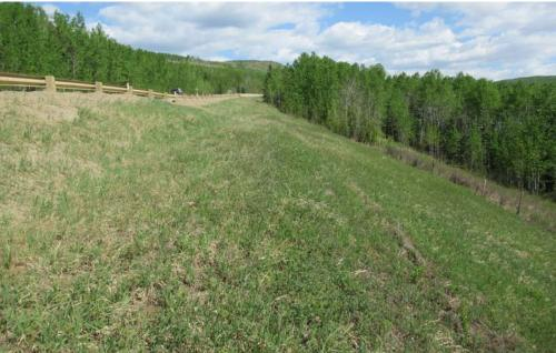
Photo 3 - Looking east along the south highway embankment, at a dip beginning to form in the embankment. Note the well grassed/vegetated sideslope. There is also a bow in the fence (not visible in the photo).
