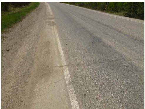
Photo 4 - Looking west at the old cracks reflecting through the chip seal, and a dip/sunken eastbound shoulder of the highway located at the east end of the site.
