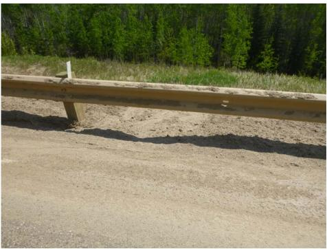
Photo 2 - Looking south at the guardrail at the west highway dip. Note the accumulated sand/gravel on the EB shoulder (~50 mm high), that channelizes runoff from the highway.
