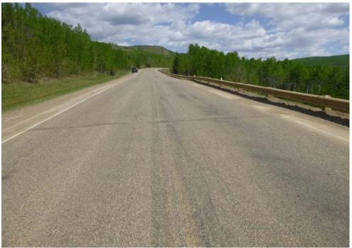
Photo 1 – Looking east along the highway from the far west end of the site. The fall, 2017 chip seal has camouflaged the cracks. Note the west dip in the road/guardrail in the background.
