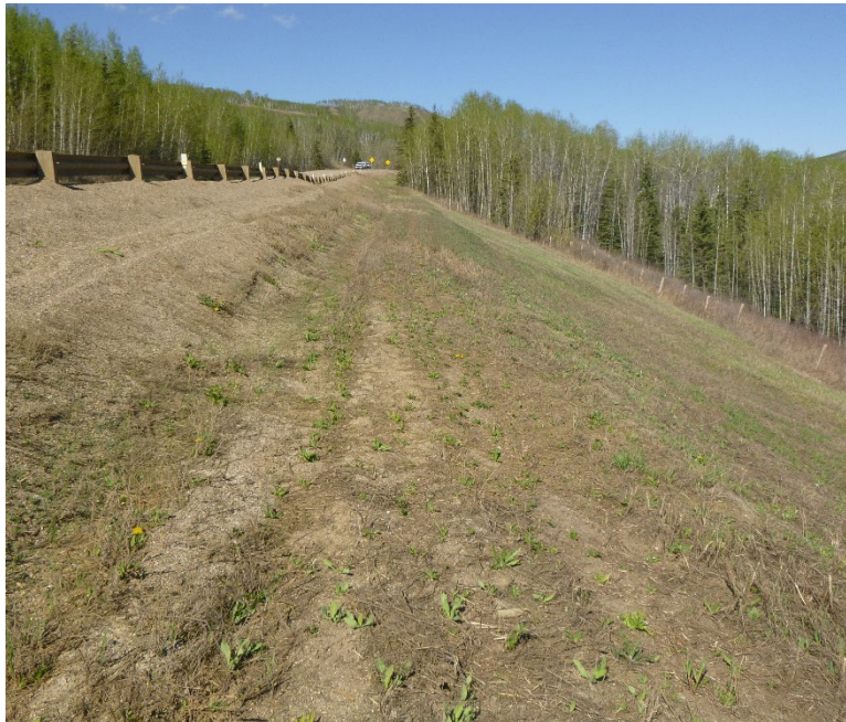
Photo 2 - Looking east along the south embankment and the bowed fenceline from the west end of the site. Note the dip in the embankment below the patched west scarp crack area.
