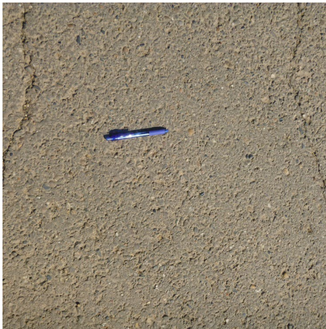
Photo 6 – Close-Up view of the two WB lane cracks reflecting through the east end scarp crack patch shown in Photo 5.
