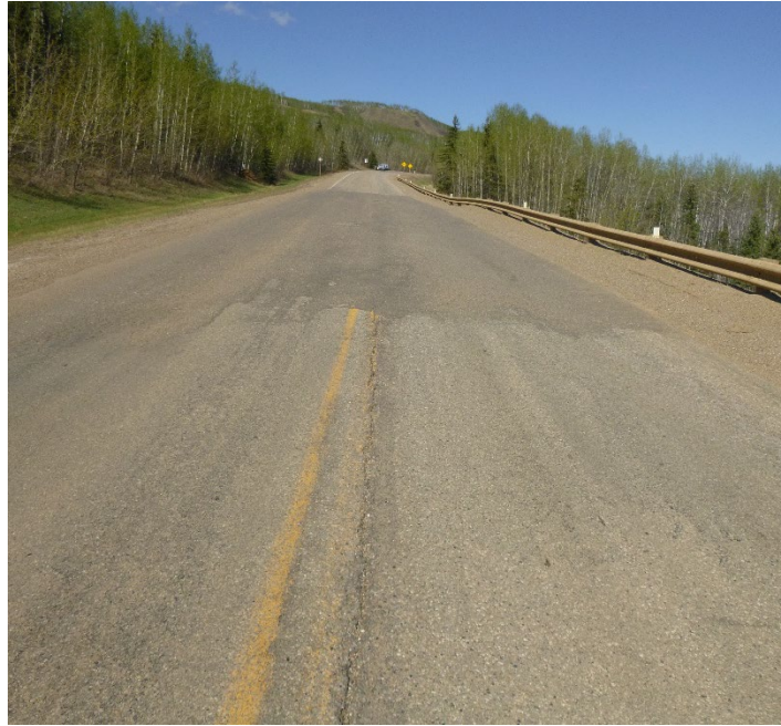
Photo 1 – Looking east along the cracked highway surface from the west end of the site. Note the fresh patch over the west end scarp crack and the dip in the south guardrail.
