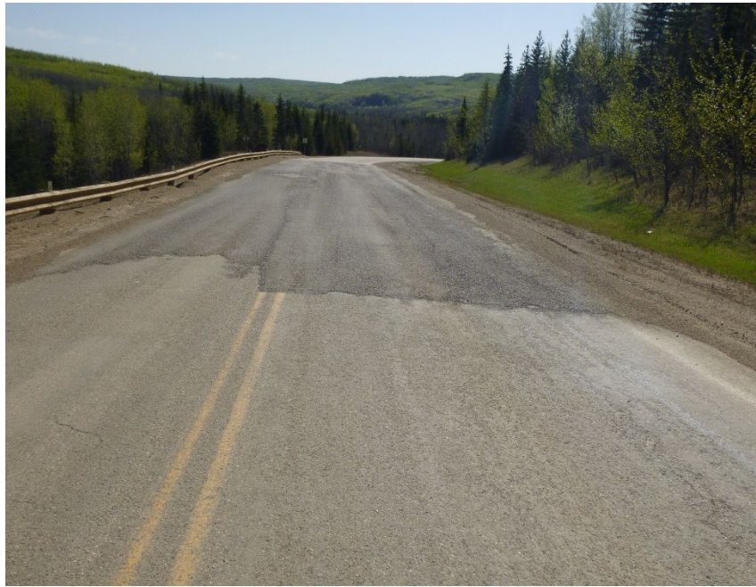
Photo 3 - Looking west at the fresh patch and the dip/sunken highway where the slide scarp crosses the west end of the site.
