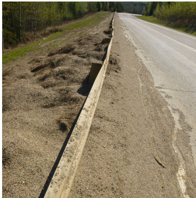
Photo 4 - Looking west along the south guardrail at the location where a broken hay bale is trapping sand along the edge of the highway between the east and west scarp cracks. Note the channelized surface runoff that has been created, and it has breached the sand build-up underneath the south guardrail and created an erosion gully in the hwy embankment slope below the dip in the highway further west.
