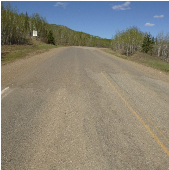
Photo 5 – Looking east at a fresh ACP patch over where the east slide scarp crosses the highway at the east end of the site.
