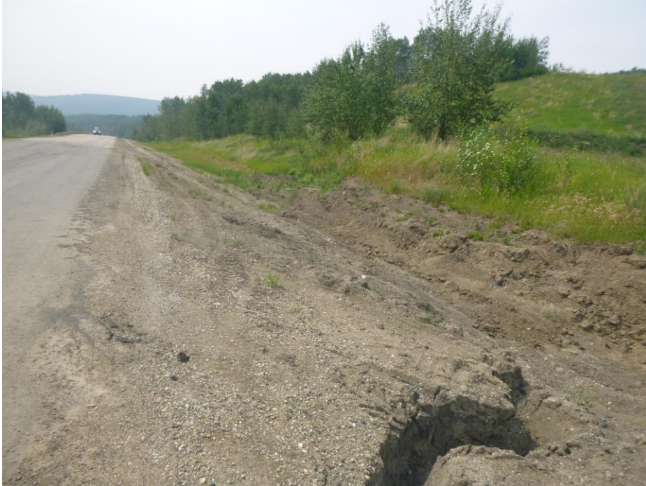
Photo 11 - Looking northwest along the main scarp from near the east edge of the highway. Note the erosion gully in the foreground.
