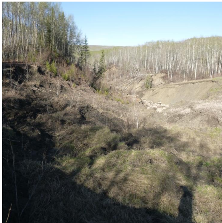
Photo 16 – Looking west along the eroded creek channel from near the twin pipes outlets.
