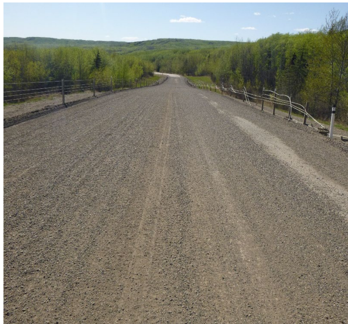
Photo 10 – Looking west along the road. Note the damaged and loose north HTCB.
