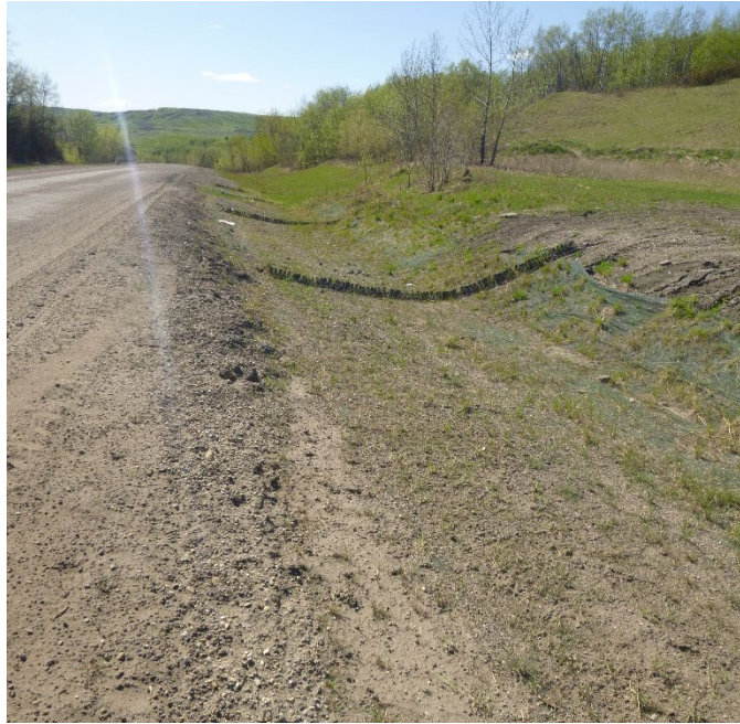
Photo 13 – Looking west along the north highway ditch at the former sagged area that had ponded water. Water was drained, the former north approach was removed and the ditch was graded and lined with TRM as part of the 2023 road surface gravel conversion project.
