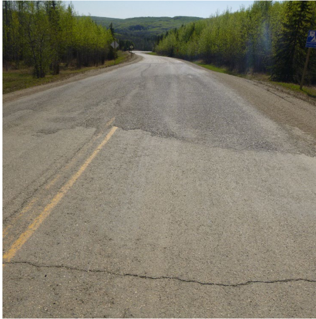
Photo 5 - Looking west at the milled/patched area over the two slide cracks first observed in 2013 that mark the west boundary of the slide on the highway.
