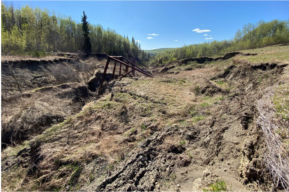
Photo 15 – Looking west along the eroded channel at the twin pipe riser inlets, eroded trash rack, and gabion remnants.
