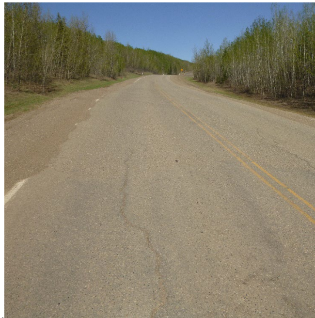
Photo 6 – Looking east at the same slide crack and scarp as Photo 5 that extends into the north ditch. Note the two settled areas along the north edge of the highway embankment.
