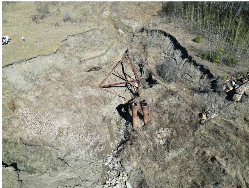
Photo 2 – UAV Looking east at the trash rack, twin culvert riser pipes, and remaining gabion remnants.
