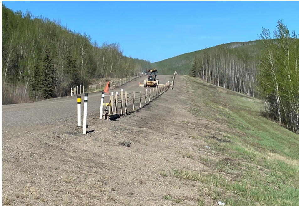
Photo 7 – Looking east just east of where a landslide crack and large dip used to be visible in the road surface and north ditch before the road surfacing was converted to gravel in 2023.
