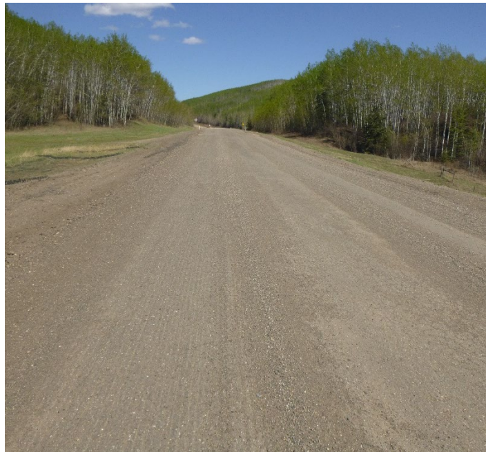
Photo 12 – Looking east along the north ditch that was re-graded and lined with TRM, across the area where the east slide crack was affecting the highway.
