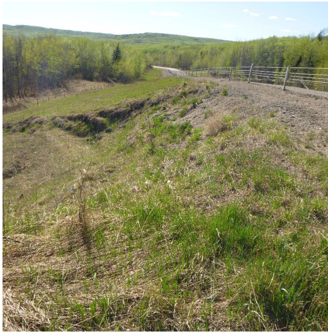
Photo 9 – Looking west along the south edge of the highway at Embankment Slump A.
