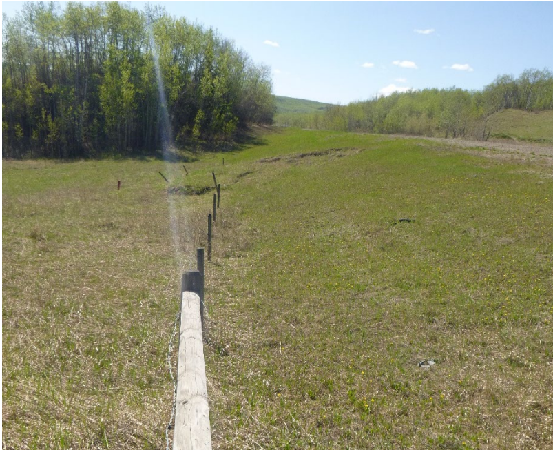
Photo 14 – Looking west at the slump in the south highway embankment sideslope at the east end of the site. Note how the toe has pushed the fence downslope.
