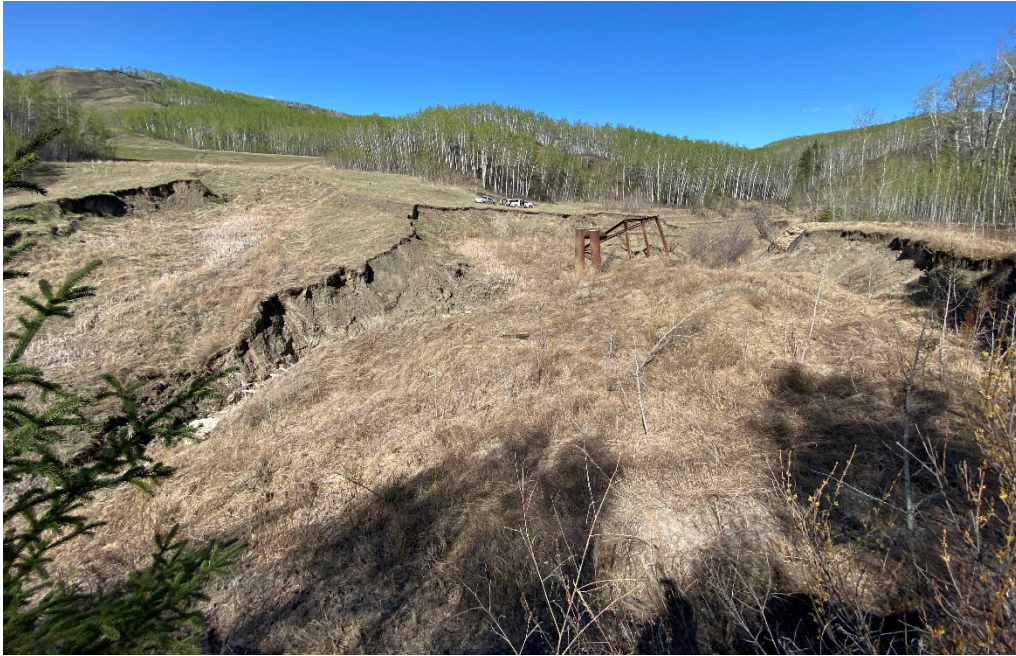
Photo 17 – Looking north across the eroded tributary channel towards the highway, at the eroded piping area (LHS), twin pipe inlets and trash rack (Center), and eroded gabion weir (RHS).
