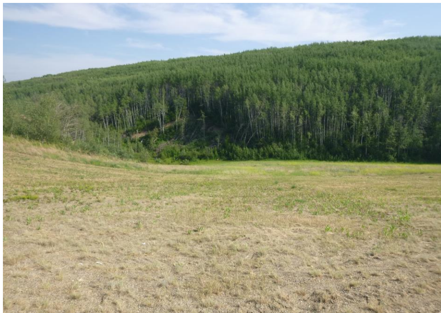
Photo 12 – Looking south at the valley slope slumping above the 1200 culvert inlet and gabion outlet area, caused by rapid drawdown of built-up floodwater.
