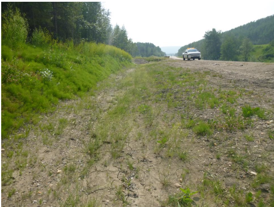
Photo 2 – Looking west along the unlined south ditch from near the west end, at the 2020 grading that took place along the south highway embankment and ditch.
