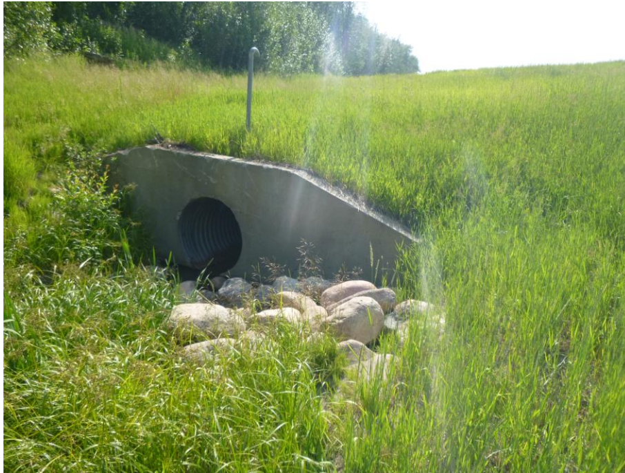
Photo 11 – Looking west at the 1200 mm CSP inlet headwall.
