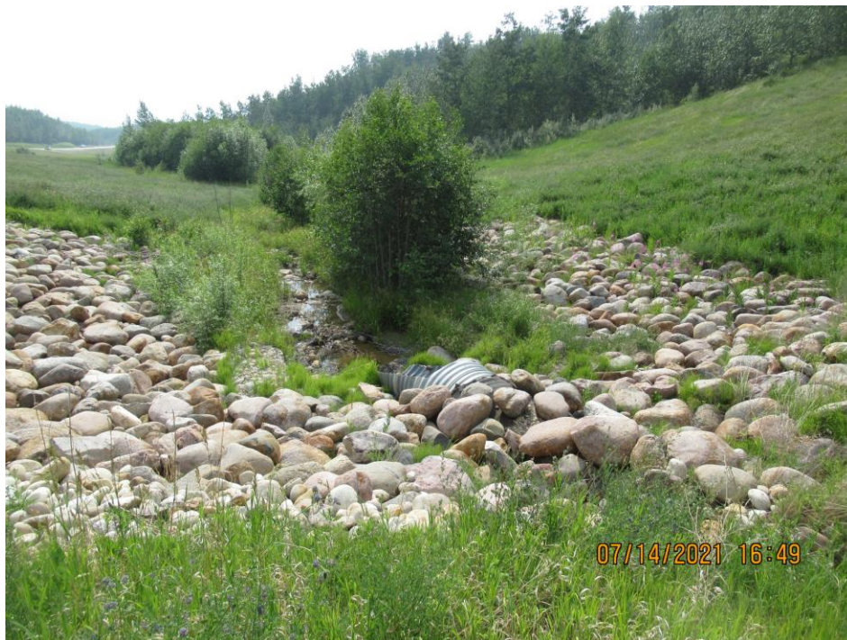
Photo 22 – Close-up view of culvert outlet, looking west.
