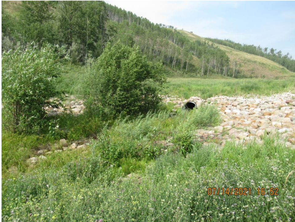
Photo 21 - Looking east at the 1200 CSP outlet area in the north channel.
