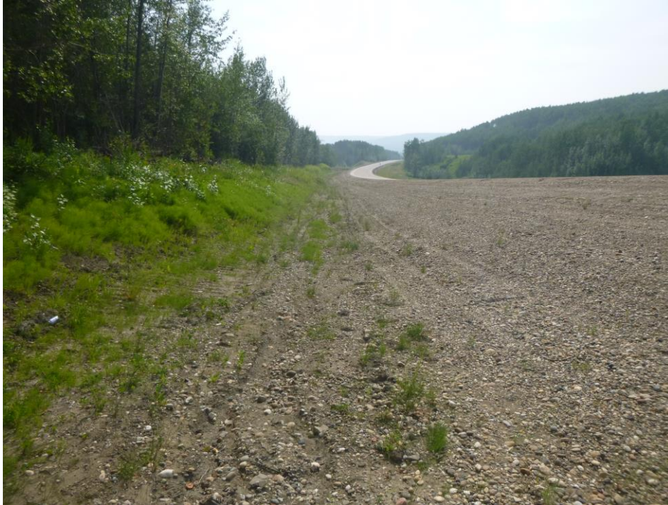
Photo 3 – Looking west along the south ditch and hwy embankment.
