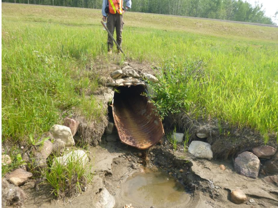
Photo 15 - Looking south at the 810 CSP outlet along the north ditch channel that was cleaned in 2020. Note the erosion scour bowl forming.
