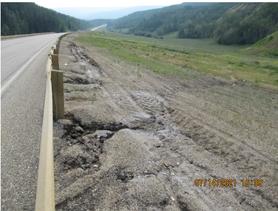
Photo 14 – Looking west at the rilling adjacent to the north guardrail (just west of the repaired rilling on the north embankment).
