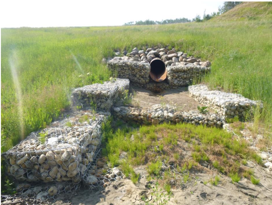
Photo 10 - Looking north at the 900 SWSP outlet and gabion outlet structure.
