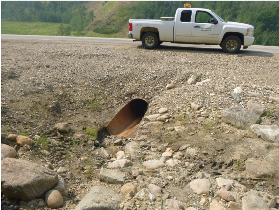
Photo 5 – Looking north at the inlet of the clean 760 mm dia. SWSP.
