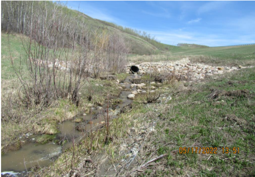
Photo 21 - Looking east at the 1200 CSP outlet area in the north channel.
