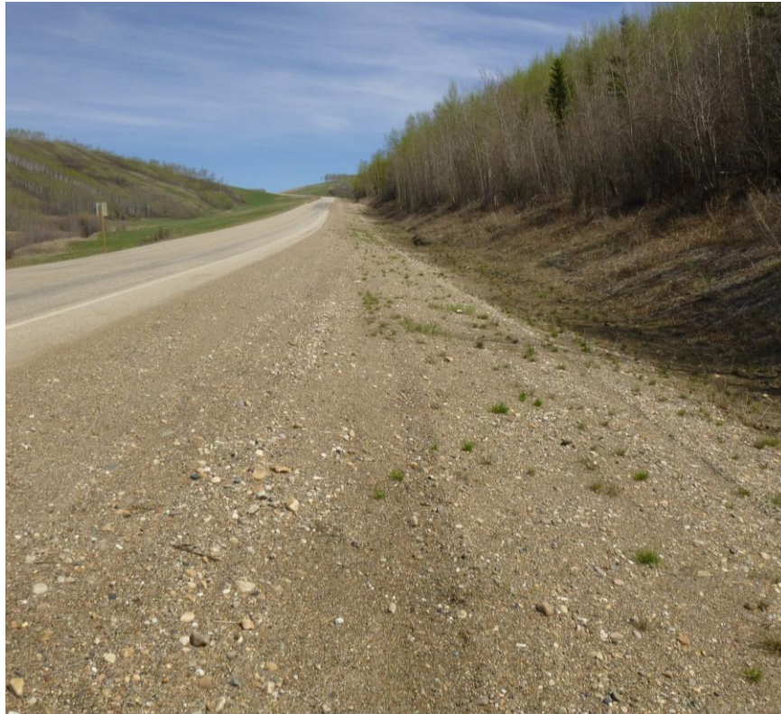
Photo 5 – Looking east along the south ditch and hwy embankment.
