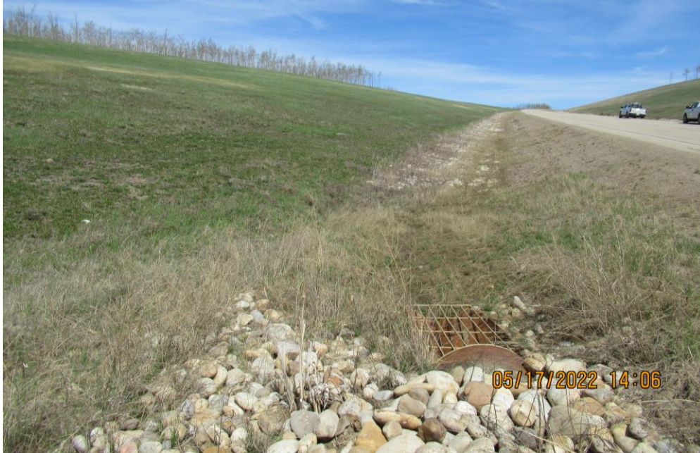
Photo 13 – Looking east along the north ditch from the north 900 mm SWSP entrance.
