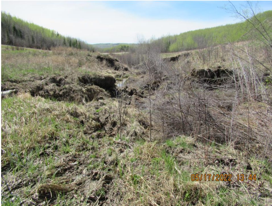
Photo 19 – Looking west (downstream) at the erosion just upstream of the 760 SWSP outlet.
