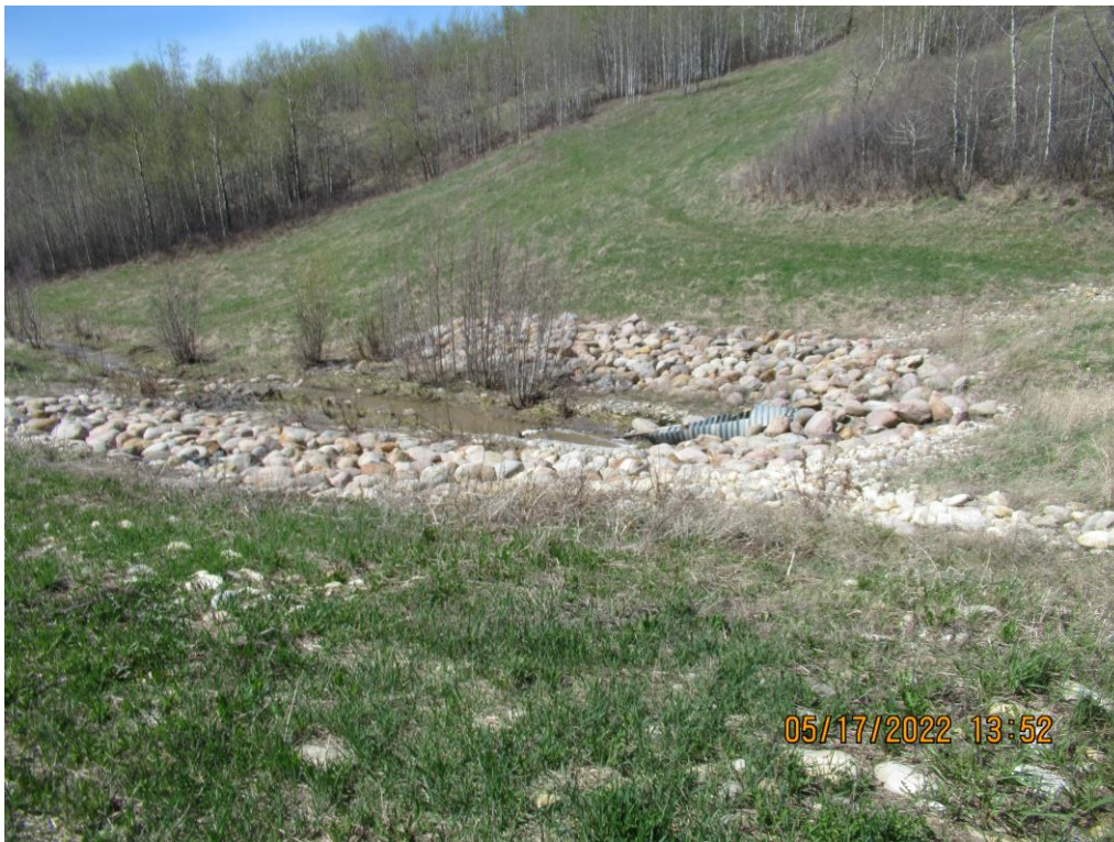
Photo 22 – Looking northwest at the 1200 culvert outlet area.
