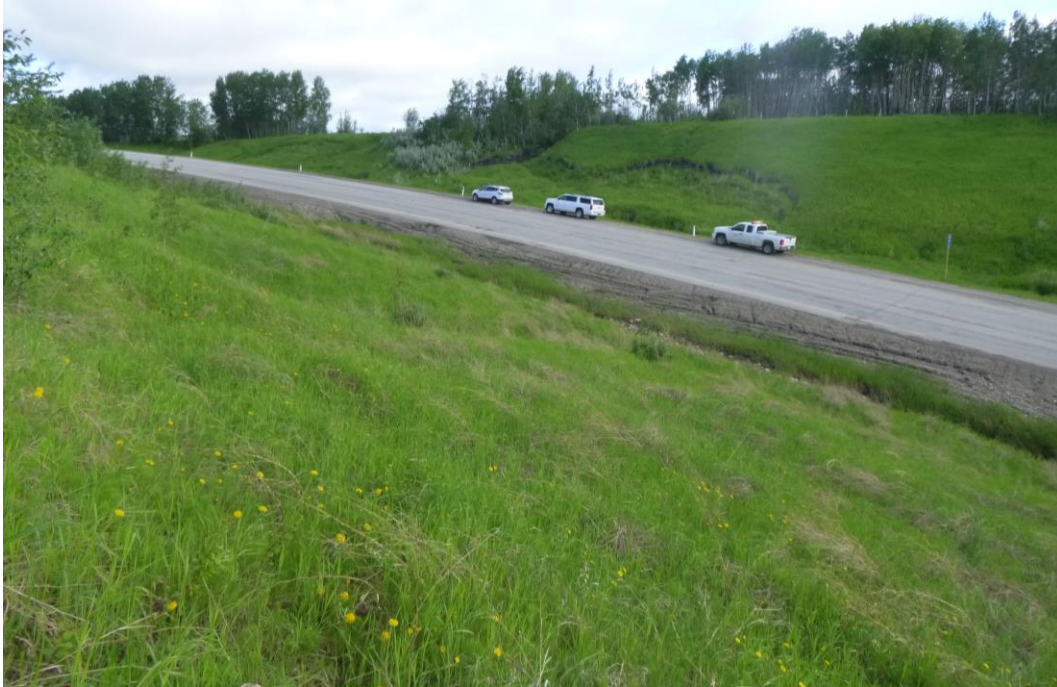
Photo 1 - Looking northwest at the west end of the north cut backslope.
