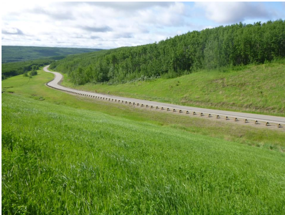
Photo 4 – Looking southeast at the east end of the south cut backslope.
