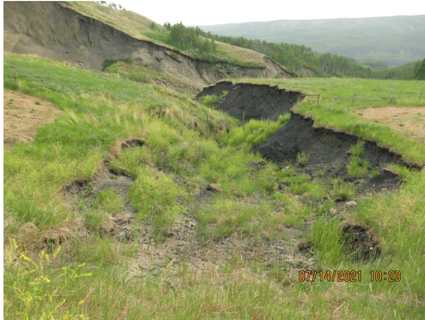
Photo 11 - Looking north from the highway at the 7 m deep erosion ravine headscarp caused by runoff from the north ditch culvert outlet. The erosion/slumping has again encroached closer to the pavement white line.
