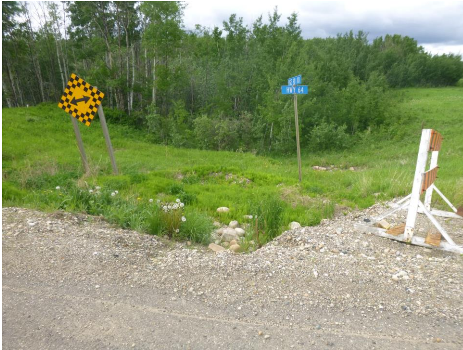
Photo 11 – Looking north from the highway overtop Slide 1.
