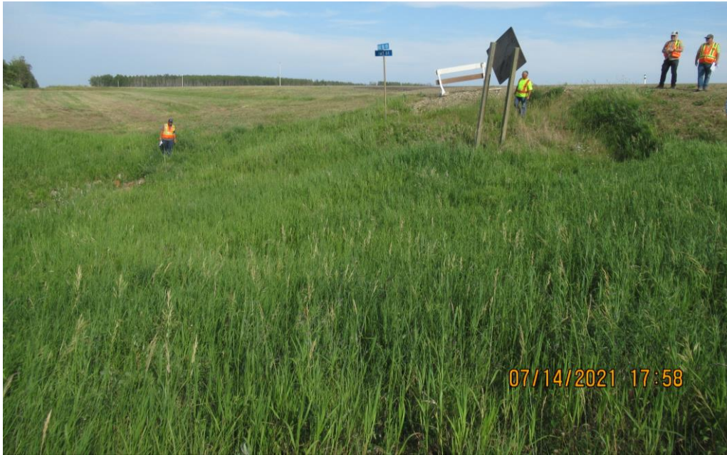
Photo 11 – Looking southeast across the Slide 1 body towards the highway.
