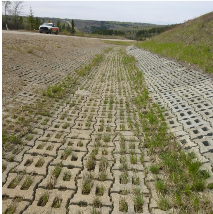
Photo 15 – Looking northwest at the ACB Matting performing well.
