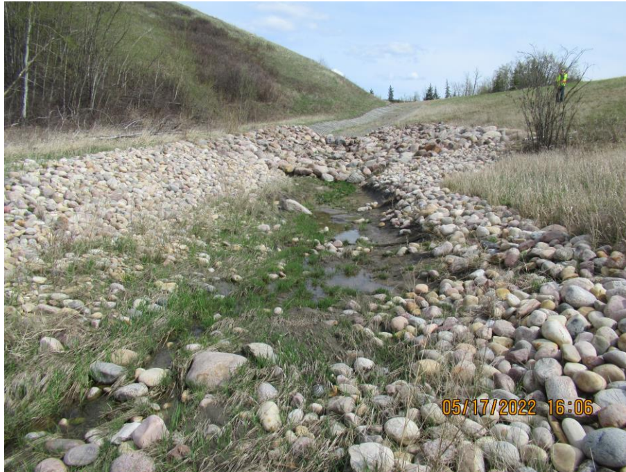
Photo 13 – Looking east at area within riprap that now has mud covering some of the riprap likely from high runoff flow events and ponding afterwards.
