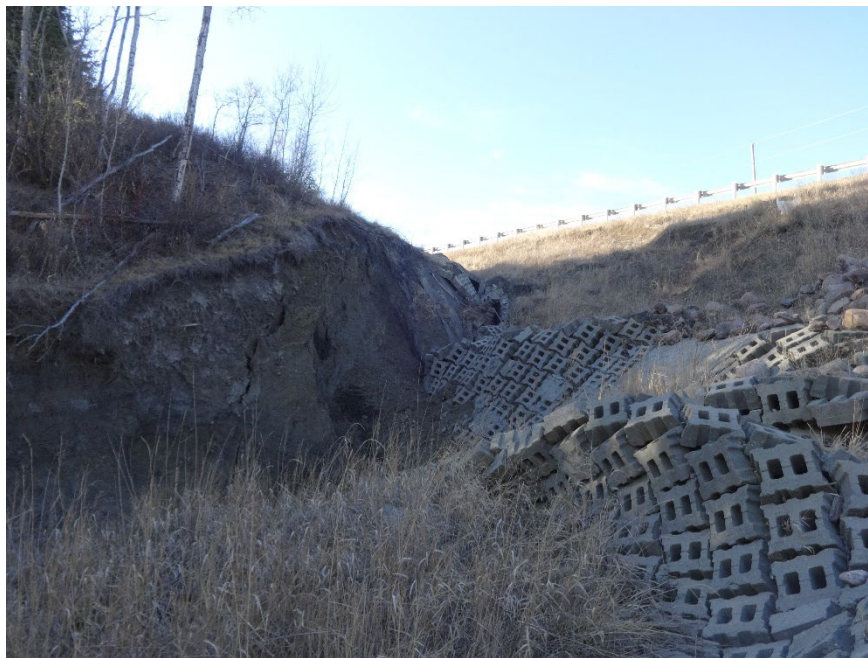
Photo 4. Looking southeast at the severe erosion through the ACB mats. Note the enlarged erosion and slide developing south of the mats.
