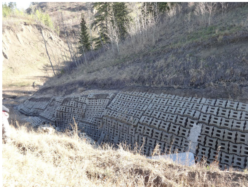
Photo 2. Looking north along the edge of the eroded ACB mat area. Note the scarp extension along the north edge of the mats.
