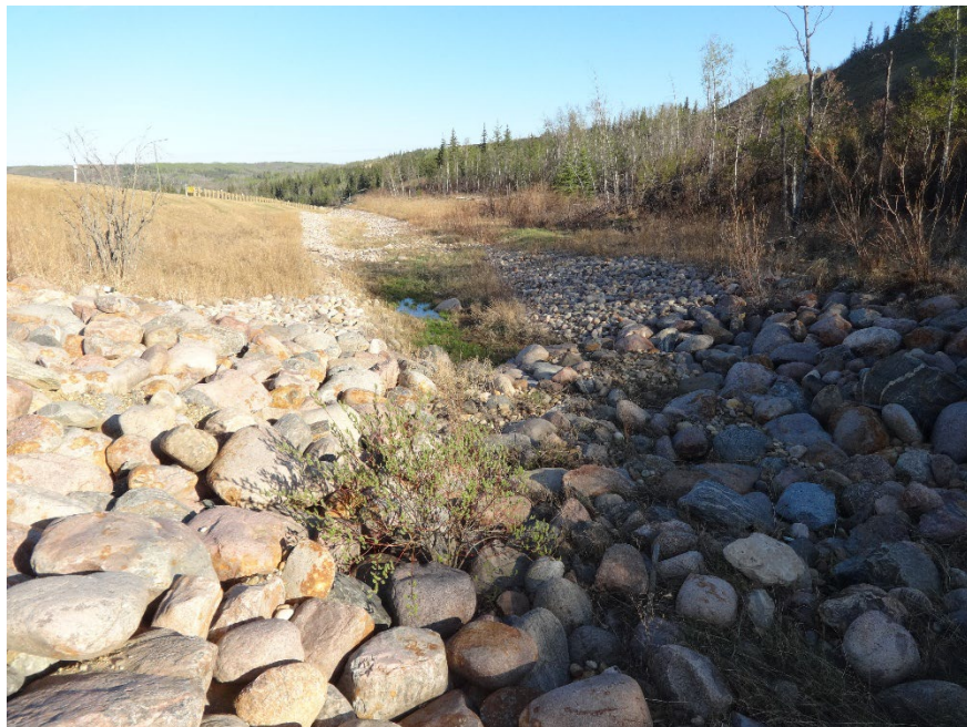
Photo 10. Looking northwest at area within riprap that now has mud and grass covering some of the riprap likely from high runoff flow events and ponding afterwards.
