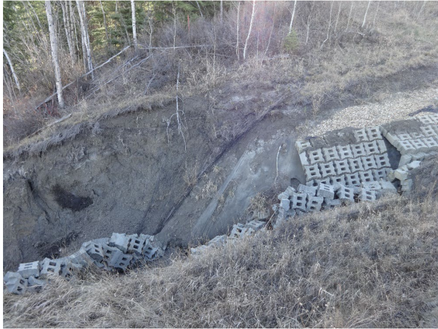
Photo 9. Looking north at the slumping and infill occurring into the channel upstream of the 1524 mm SWSP culvert inlet.
