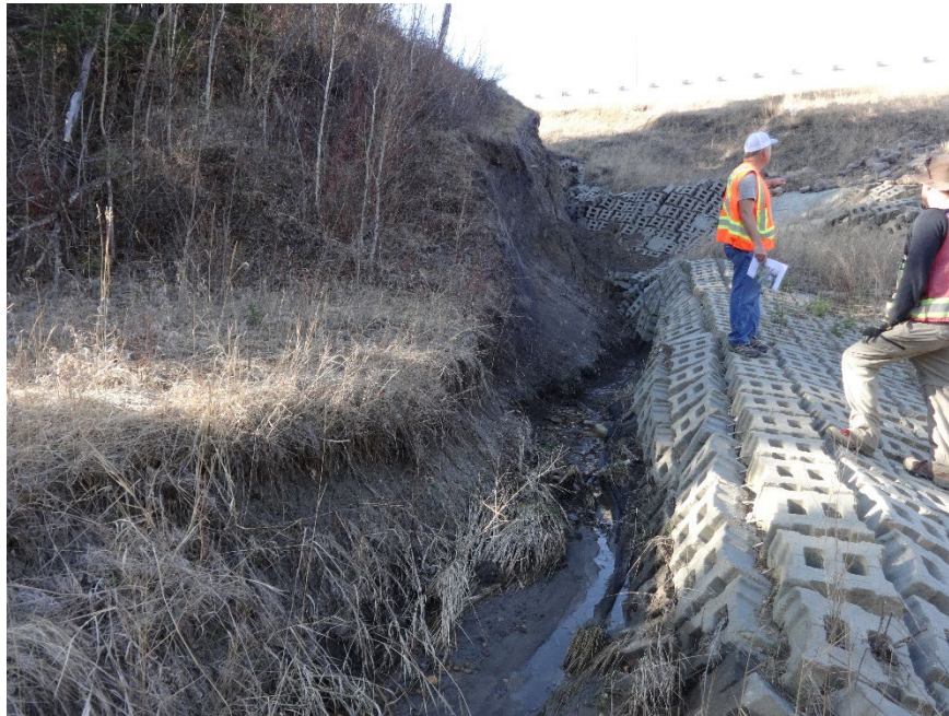
Photo 5. Looking southeast along the east edge of the eroded ACB mats. Here the mats have slid down into the deeply eroded channel and water flows along here.
