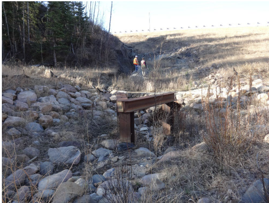
Photo 8. Looking southeast at the culvert inlet, trash rack and eroded ACB mat area leading to it.
