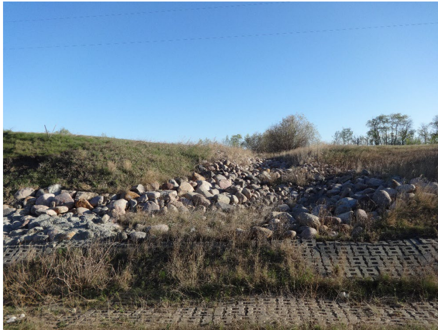
Photo 15. Looking north at where riprap was previously placed, appears to be in good condition.
