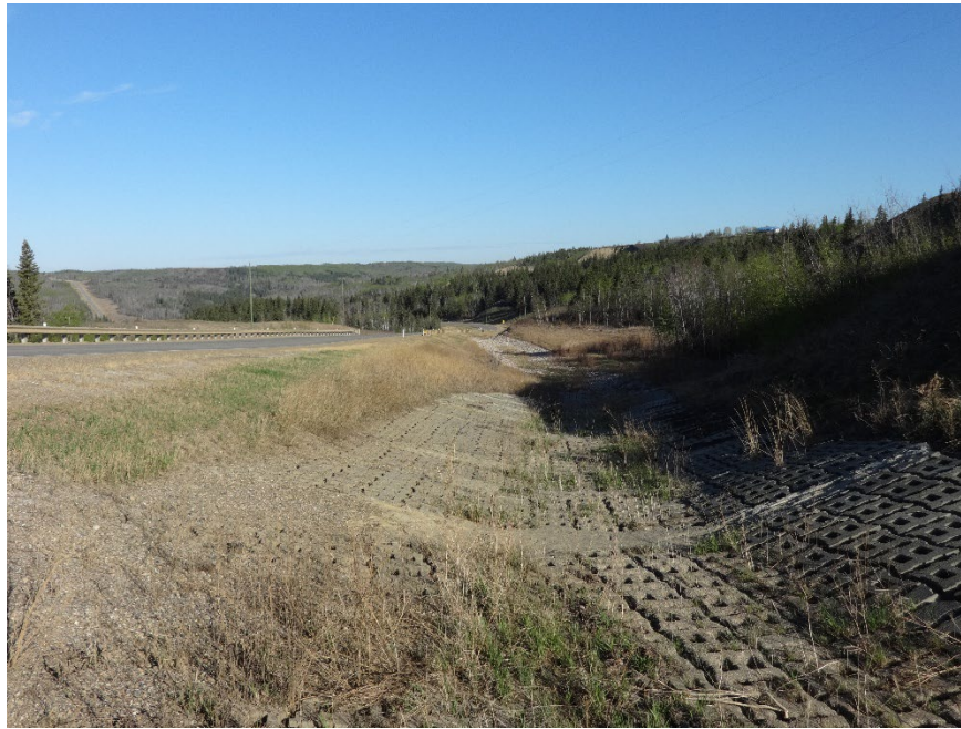
Photo 11. Looking northwest at the ACB Matting that was previously grouted.
