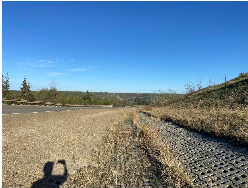
Photo 13. Looking northwest at the ACB Matting performing well and previously had some willows growing out of them which were cut.
