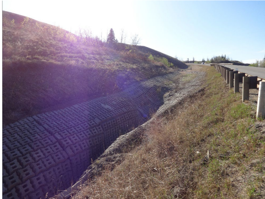
Photo 1. Looking east along the beginning of the eroded ACB mat area north of the highway.
