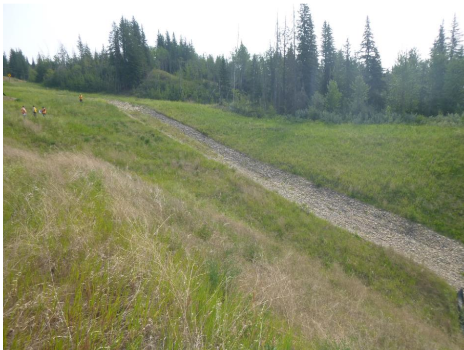
Photo 6 – Looking north along the TRM ditch channel of PH077-2.
