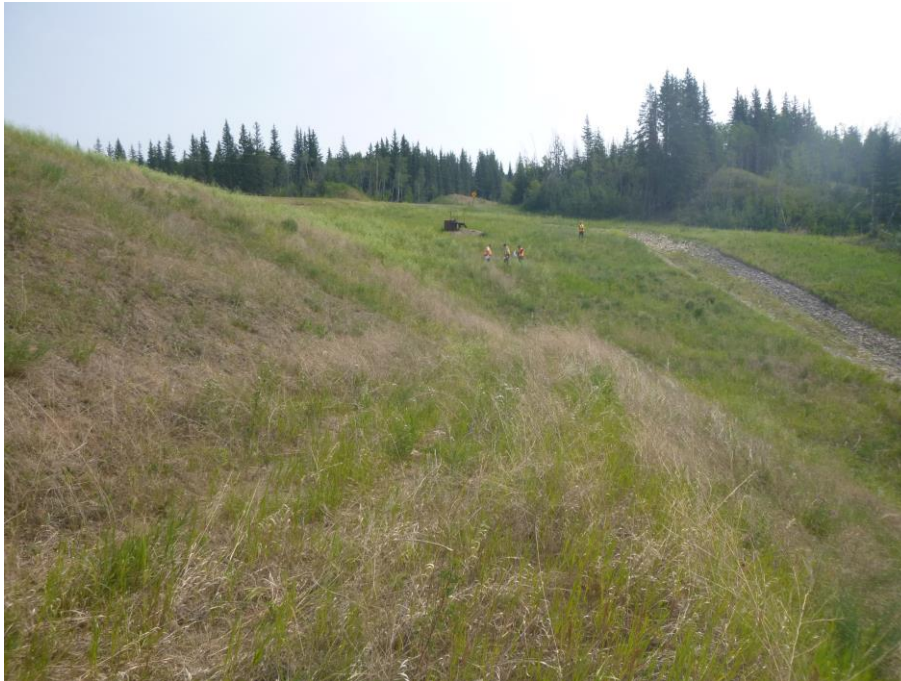
Photo 7 - Looking east along the south hwy embankment and southeast ditch drainage channel of PH077-2, Hines Creek.
