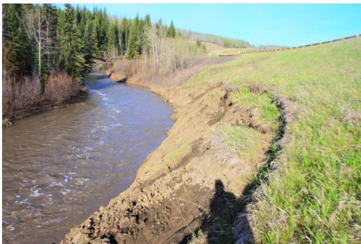
Photo 2 – Looking west at the fresh toe slumping above the creek at PH077-1 in the south highway embankment.
