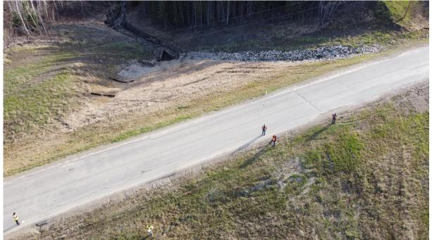
Photo 13 - Looking north from drone at infilled channel leading into the culvert inlet north of the highway at PH077-2.
