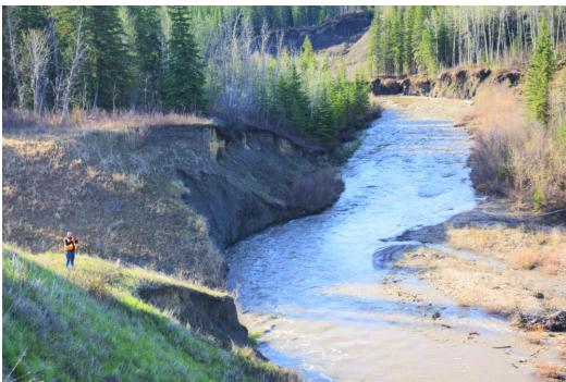
Photo 8 - Looking southeast at the river bank slumping near the culvert outlet area of PH077-2.
