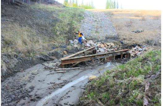
Photo 10 – Looking south at the culvert inlet area of the north embankment of PH077-2. The trash rack and culvert inlet were half full of debris and silt.
