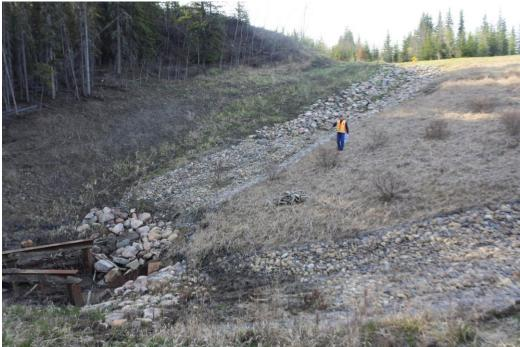
Photo 9 – Looking south at the northeast ditch crotch of the north embankment of PH077-2. In 2021 the riprap protection had been extended further upslope.
