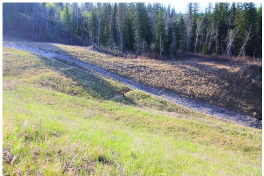
Photo 6 – Looking east at riprap swale into the gabion mattress channel of PH077-2.
