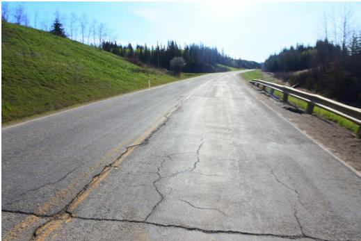
Photo 4 - Looking east along the highway at the crack/dip in the highway above the Slide at PH077-1.
