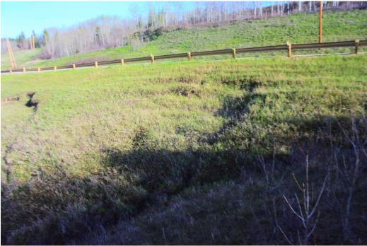
Photo 3 – Looking north upslope at the older slide scarp adjacent to the highway at PH077-1.
