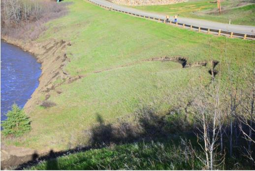
Photo 5 - Looking west at new slump that developed west of the knob hill.
