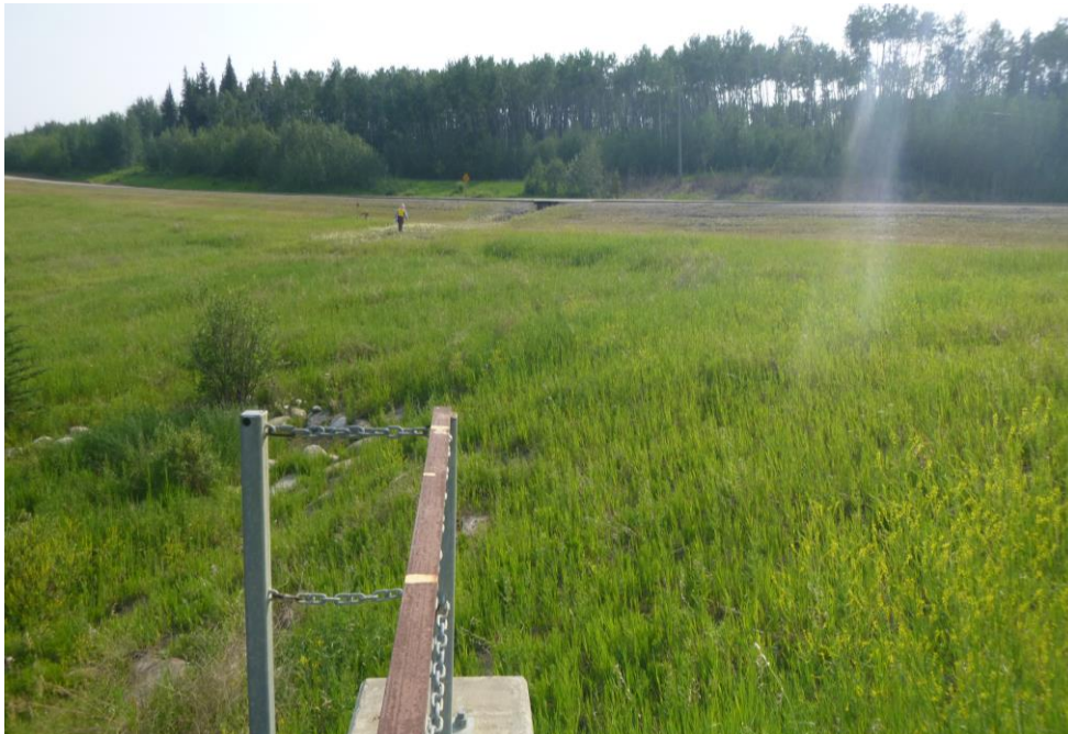
Photo 10 - Looking southwest across Slide Site 1 from northeast of the river (Site 4 is on the left-hand side). Note the grassed over slide scarp parallel to the highway.
