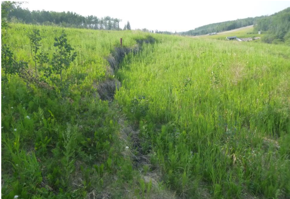
Photo 8 – Looking northwest along the fresh extended slide scarp/crack of Site 2, from just north of the most active portion of the slide.
