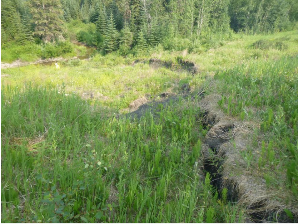
Photo 7 - Looking southeast across the most active portion of the slide block at Site 2 adjacent to the river, and the adjoining scarp extension northwards.
