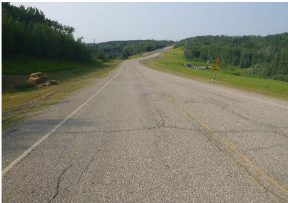
Photo 14 – Looking north along the highway at the pavement separation area across Site 4 and towards Site 1.
