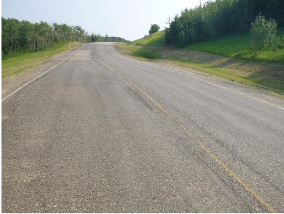
Photo 3 – Looking south at the slide scarp crossing the highway at Site 2. Note the dip in the highway, and the settled west ditch which was dry this year.
