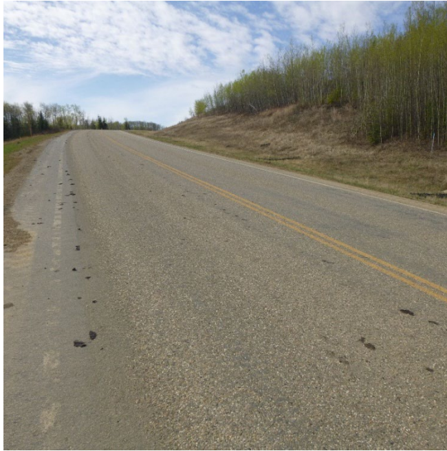
Photo 3 – Looking south along the hwy and west ditch of Site 2. Note the old, grassed-over backslope slumps, and a predominant ungrassed area where the 2023 construction detour existed.
