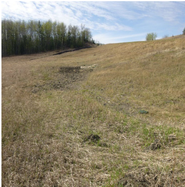
Photo 4 – Looking south along the east sideslope at steady slight seepage from the 2023 subdrain outlet constructed beneath the new Lightweight Geofoam fill at Site 2.
