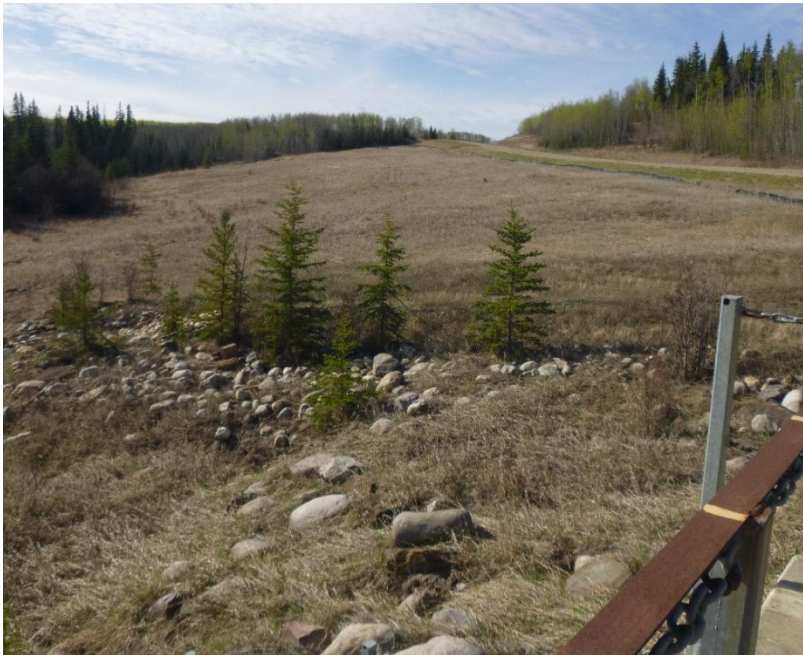
Photo 7 – Looking south across the 2023 SWSP and outlet (Site 1). Note the dipped ground surface on the RHS of the photo overtop the Site 1 slide.
