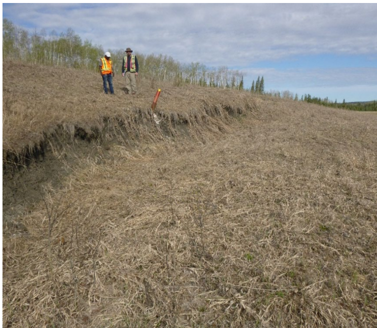
Photo 6 – Looking northeast along the active slide scarp/crack of Site 2, from just north of the most active portion of the slide.
