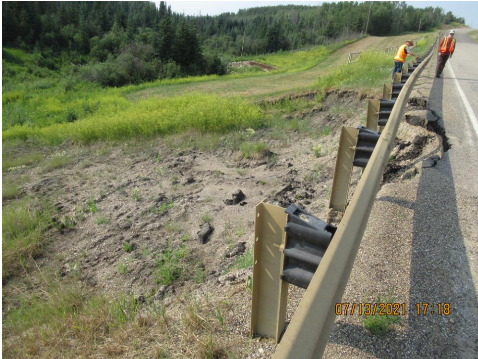
Photo 1 – Looking north along the highway south of the upper pile wall at the landslide that developed at Site #3.
