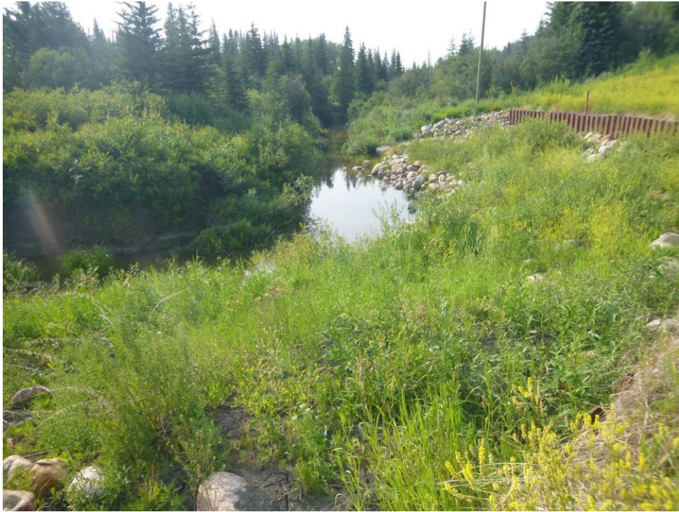
Photo 11 – Looking northwest at the lower pile wall area, Site 3.
