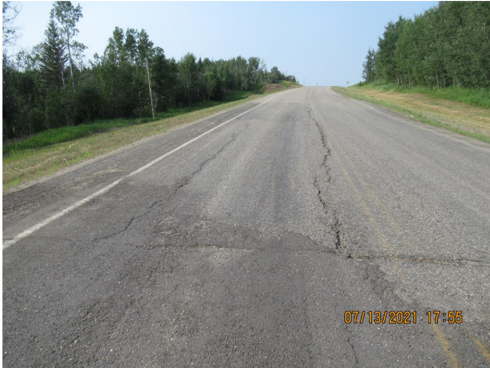
Photo 17 - Looking north along the highway at the additional subsidence in the NBDL and shoulder at Site 5.
