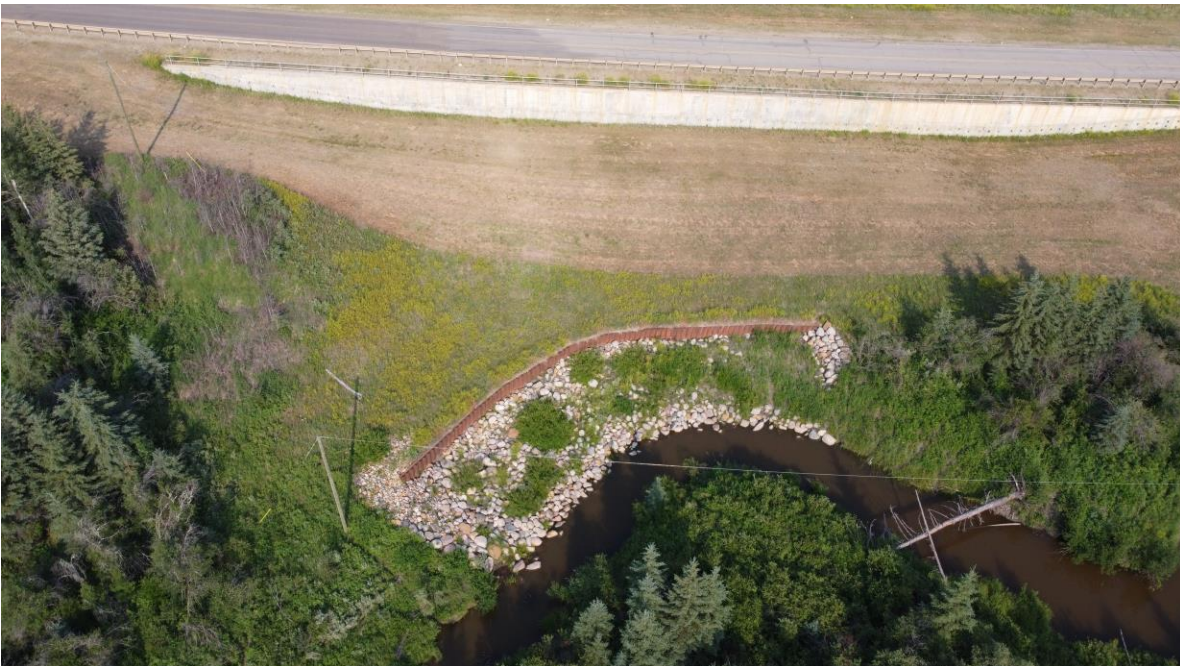
Photo 6 – Drone photo of the upper and lower pile walls at Site 3.
