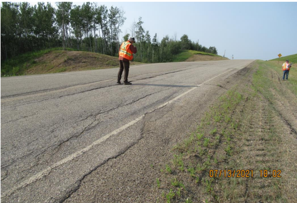
Photo 20 - Looking northwest from the east highway edge at where the slide scarp crosses the highway at the north end of Site 6.
