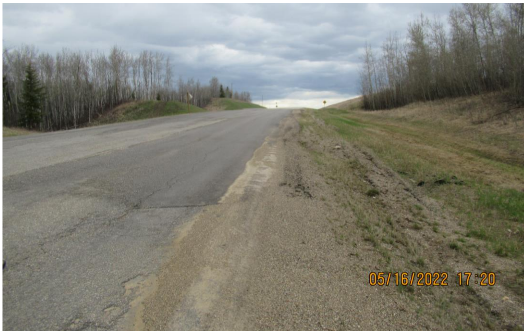
Photo 14 - Looking north along the east highway edge at where the slide scarp crosses the highway at Site 6.
