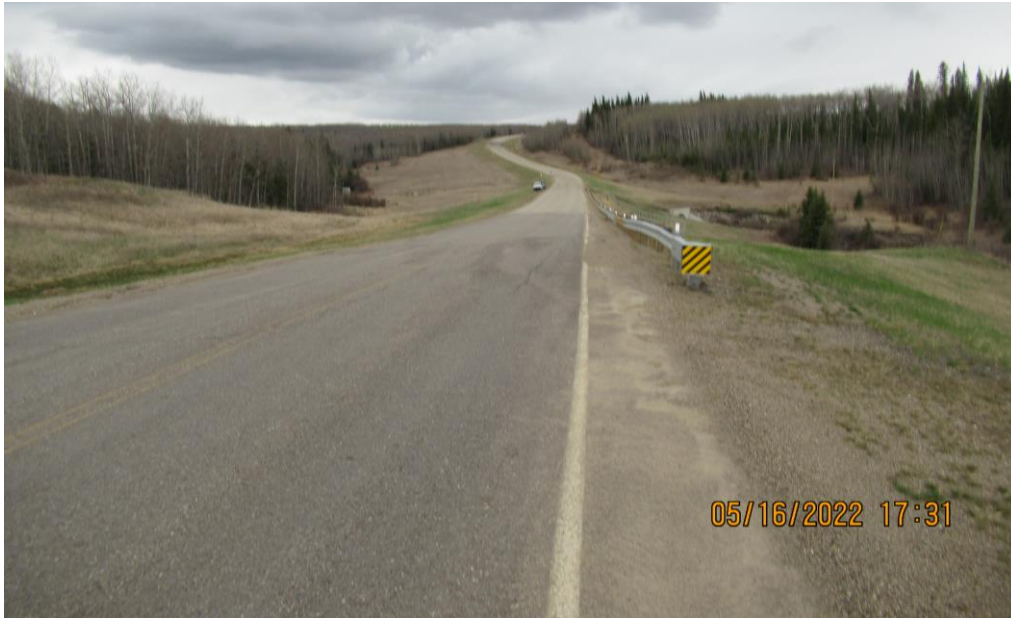
Photo 11 - Looking south along the highway from just north of the hump in the patch near the north end of the pile wall at Site 3. Note the new Impact Attenuator.
