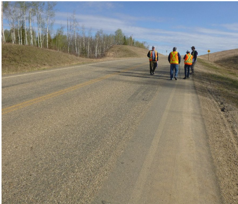
Photo 12 - Looking north along the east highway edge where the slide scarp crosses the highway at Site 6.
