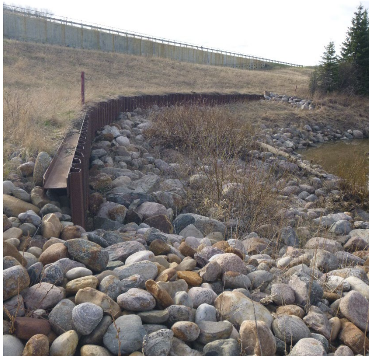
Photo 7 – Looking south along the lower pile wall, riprap, and river at Site 3.
