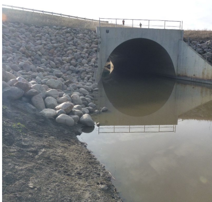
Photo 3 – Looking southeast at the slide repairs and the arch culvert outlet area at Site 3.
