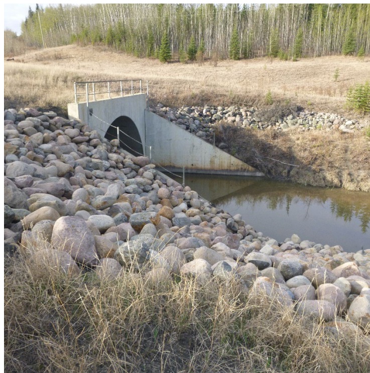
Photo 2 – Looking south at the lower slide repairs and arch culvert outlet at Site 3.
