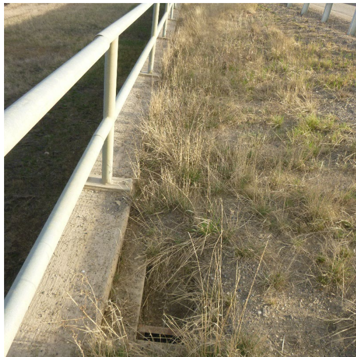
Photo 4 – Looking north at the top of pile wall gutter drain and loose cover plate at site 3. This needs to be maintained.
