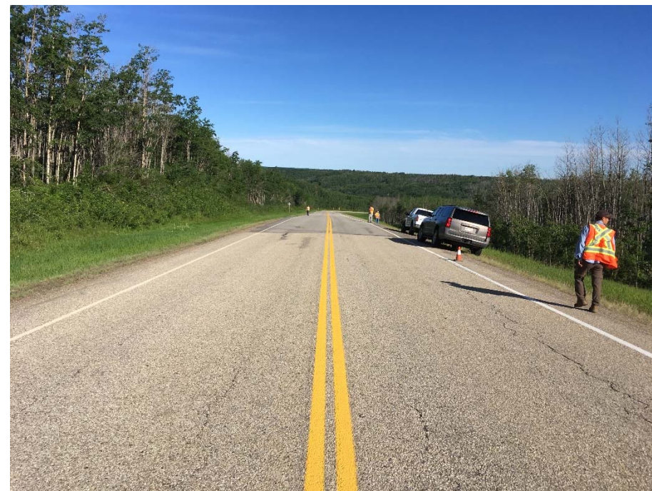
Photo 1. Looking southeast along Hwy 733.
